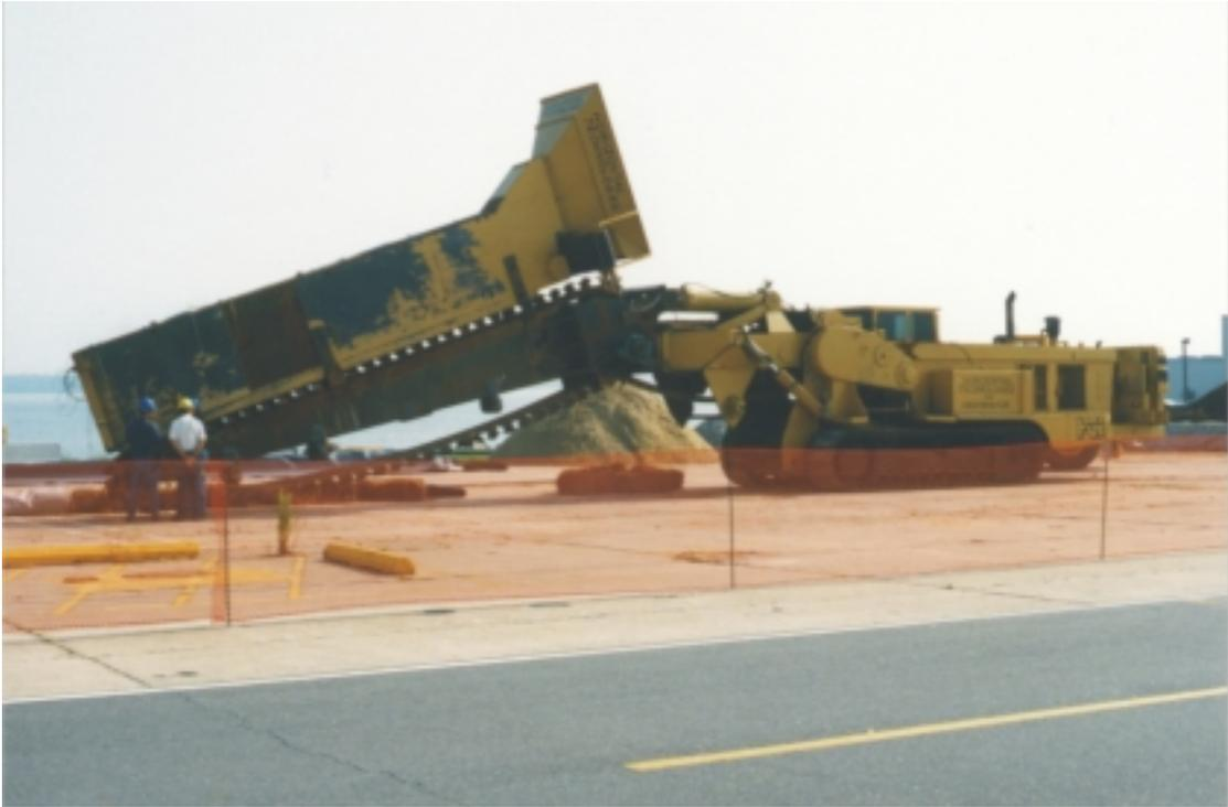
**Figure 55.** Trenching machine used to install the 7.3 m deep, 0.6 m wide granular iron barrier.
