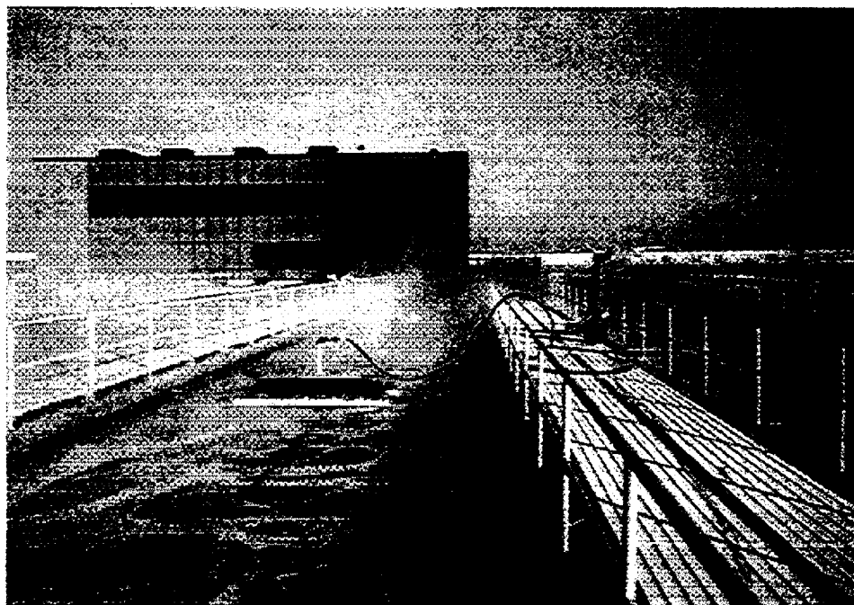
FLEXIBLE MEMBRANE OFF-GAS COLLECTION HOOD
