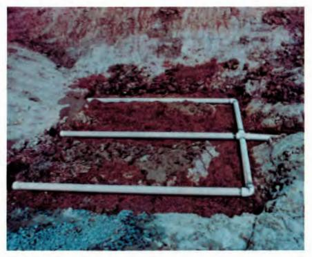
The underdrainage system, which drains seepage from the bottom of the pond and promotes dewatering of the waste (pipes may be spaced 100 ft or more in an operational site)
