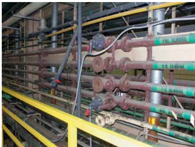
Figure 2.6 Single Pass DSS – Sampling Ports
