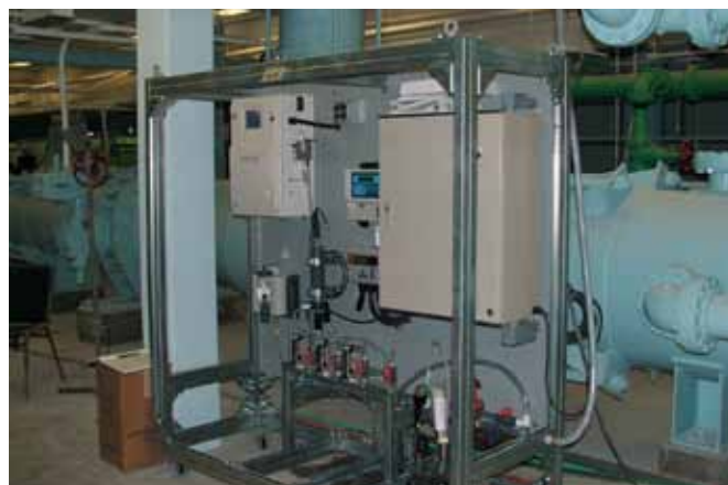
Figure 2.13 First Pilot Utility - Water Security Initiative Instrument Panel Type B
