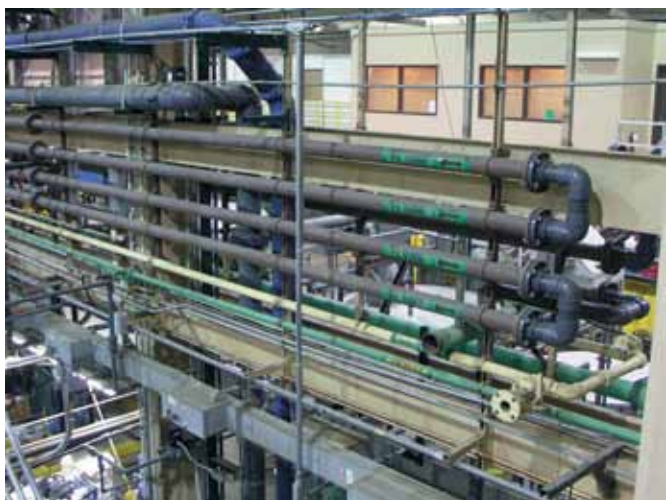
Figure 2.5 Single Pass DSS – Connecting Pipe Elbows
