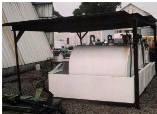
Figure 2.8 Containment structure for fuel tanks help prevent spills.
