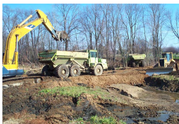
Figure 2.4 Removing sediment from the flood pool (Brate, 2004)
