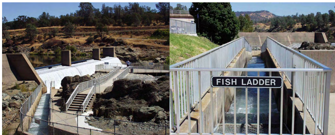
Figure 2.9 Fish Ladder at Feather River Hatchery, Oroville Dam, CA (Feather River, n.d.)
