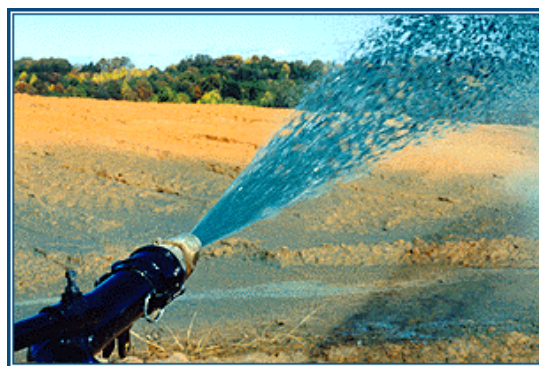
Figure 2.5 Hydroseeding (Conwed Fibers, n.d.)
