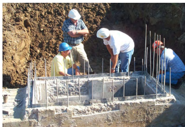
Figure 2.2 Construction on concrete riser (Brate, 2004)
