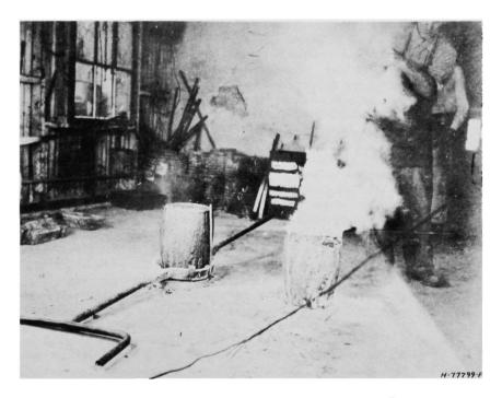
Figure 5. Transfer crucibles, with cover and without.5
