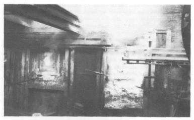
Figure 12. Fume loss at furnace doors resulting from insufficient gas volume in dust collection system.
