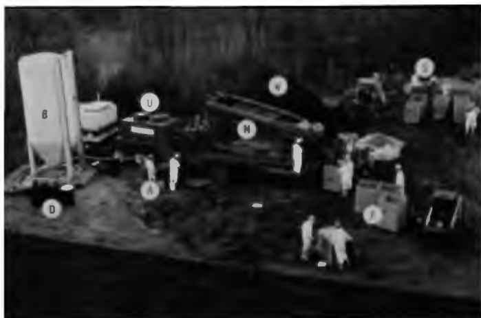
A - Proprietary additives B - Portland Cement supply D - Drums containing oily sludge F - Forms for treated waste monoliths M - Mixer S - Sample preparation U - Urrichem supply W - Filter cake waste pile
