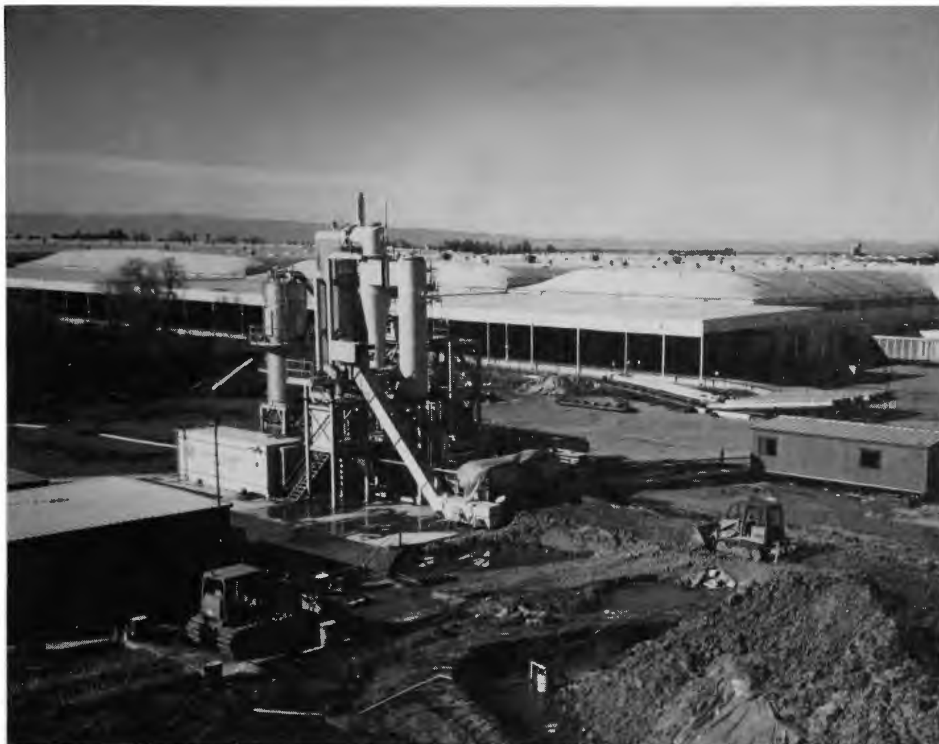
Figure 4 36-in. Diameter Transportable CBC at Stockton Site Leaking Underground Storage Tank Remediation Photo
