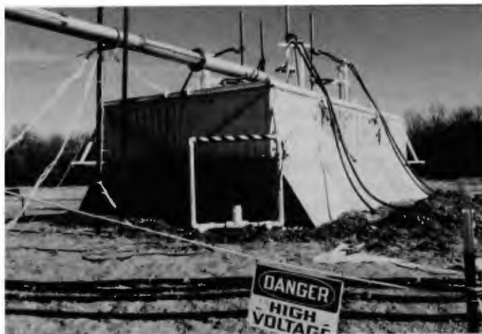
Figure 6 Off-Gas Containment And Electrode Support Hood
