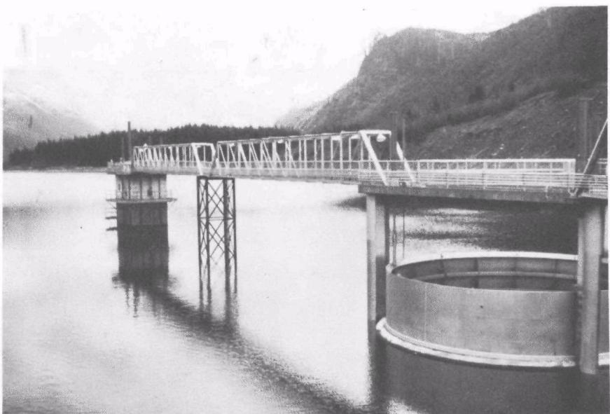
Figure B1-1. Ring gate and intake tower on South Fork Tolt Reservoir.
