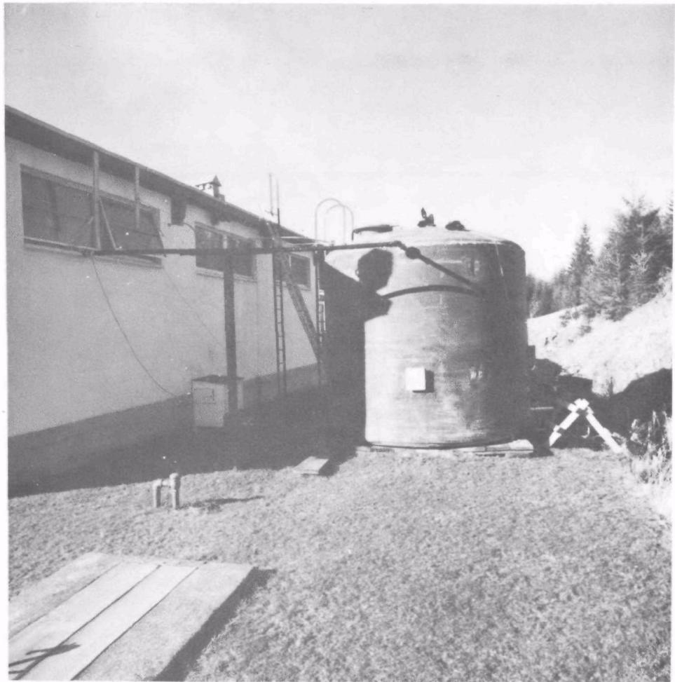
Figure Bl-14. Backwash water storage tank.
