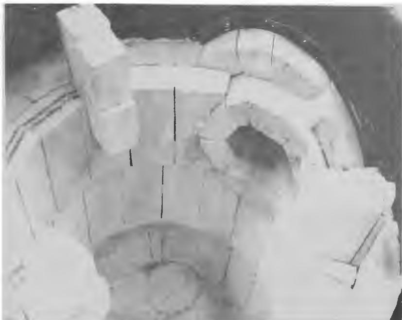
Figure 2. View through centrifugal separator and glass/fly ash reservoir during construction showing (from steel wall inward) fibrous insulation, 2000 F and 2600 F insulating brick prior to refractory cement and glass coating. Three notched insulating alumina bricks mounted on end are shown in place to support the lower two glass coated ceramic discs.
