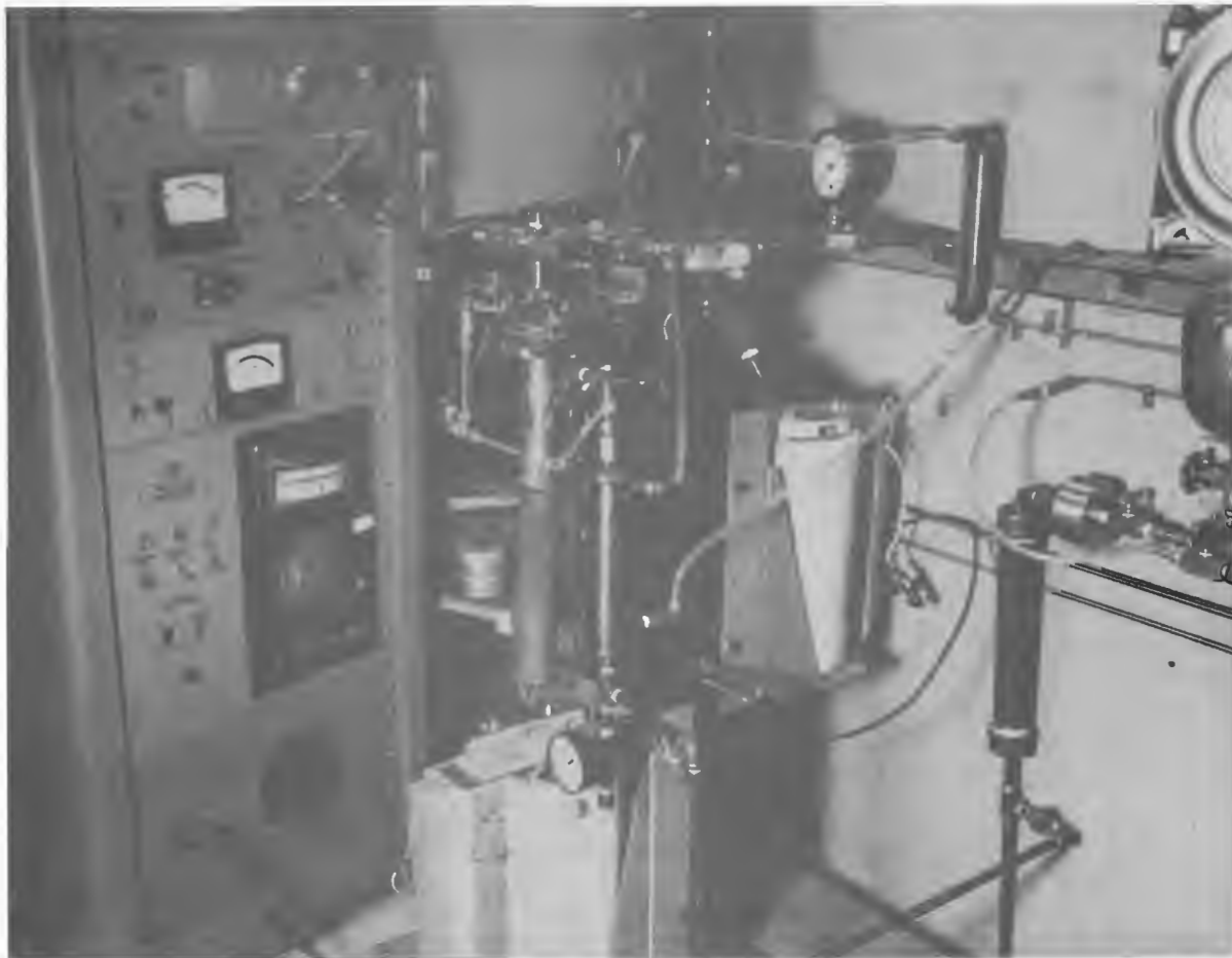
Figure 10. Fluidized-bed batch reactor system.
