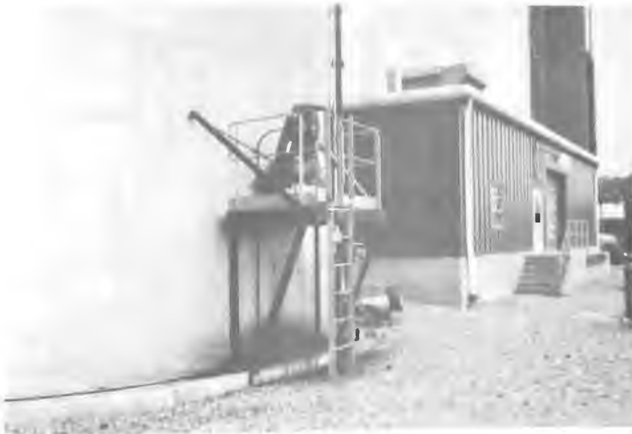
Figure 2. Process Surge Tank with Side Entering Mixer
