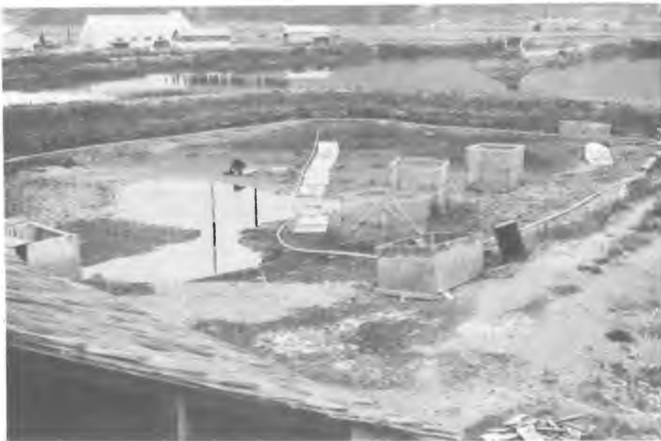
Figure 5. North Pond during pond modification, summer 1973, showing retaining wall and air line at base.
