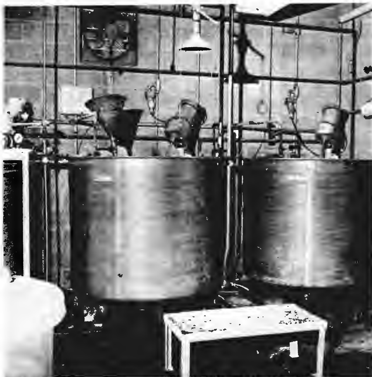
Figure 10. Alum and Polymer Solution Tanks and Metering Pumps.
