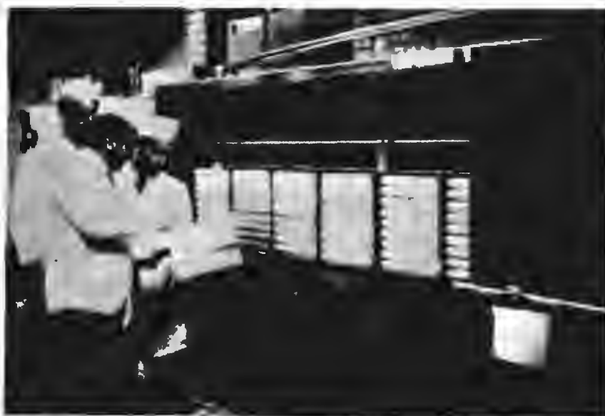
Figure 5 Pilot Plant Sanitary Cabinet Housing Ultrafiltration Membranes
