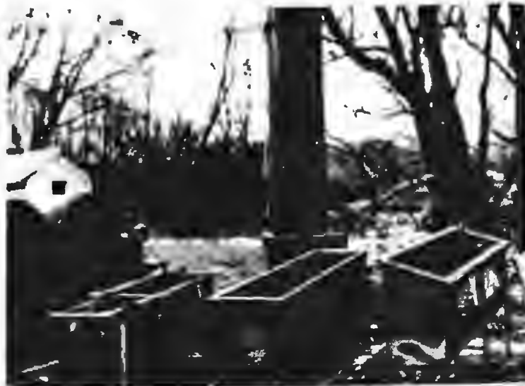
PRIMARY SETTLING TANK (LEFT) TWO BATCH SECONDARY SETTLING TANKS (RIGHT)
