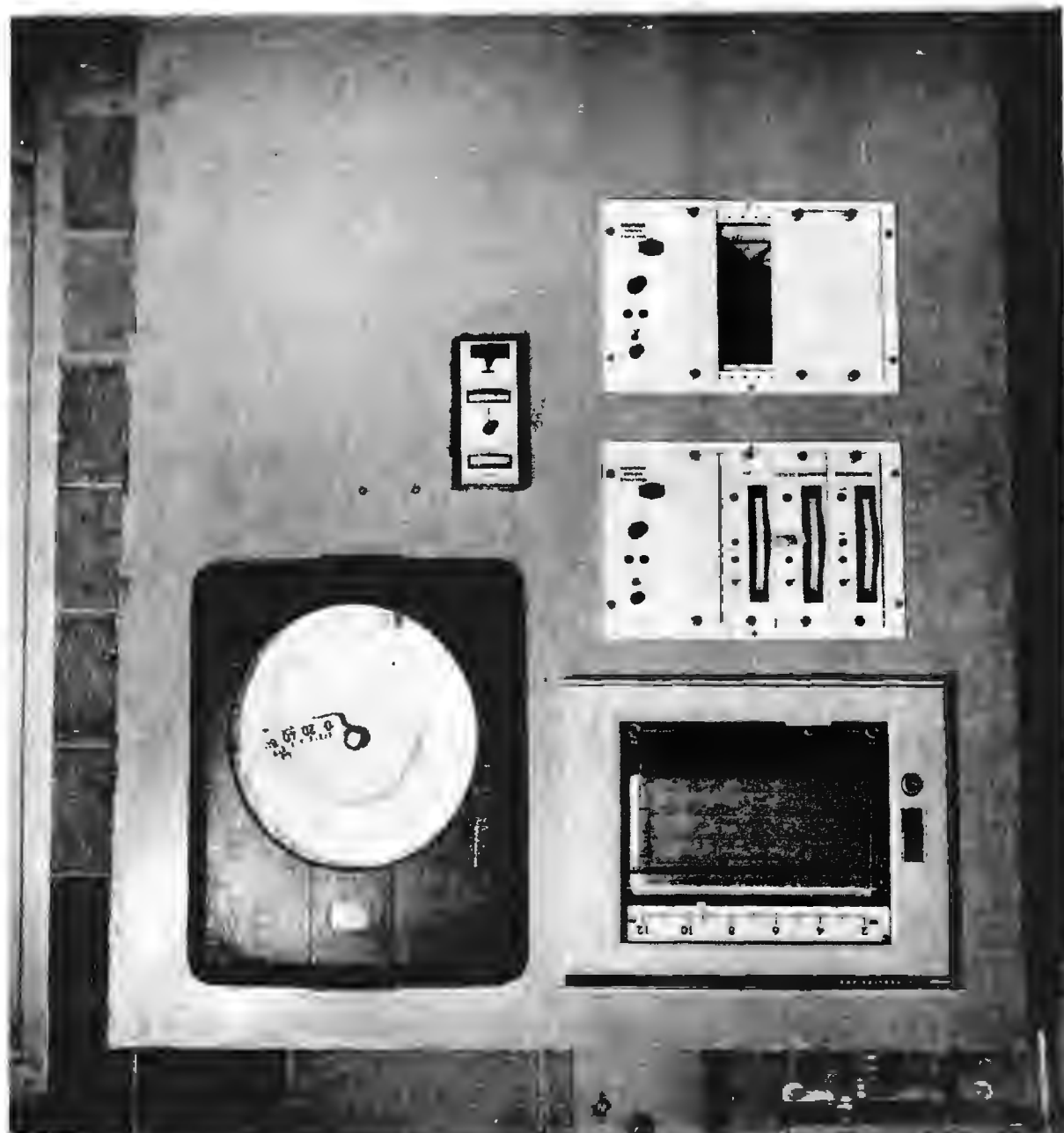
Figure 3. Instrument Panel, with Temperature, Dissolved Oxygen, Turbidity, and pH Indicators (left middle) and Recorder (top left), Magnetic Flowmeter Recorder (top right), and Controller for Acid Pump (lower right).
