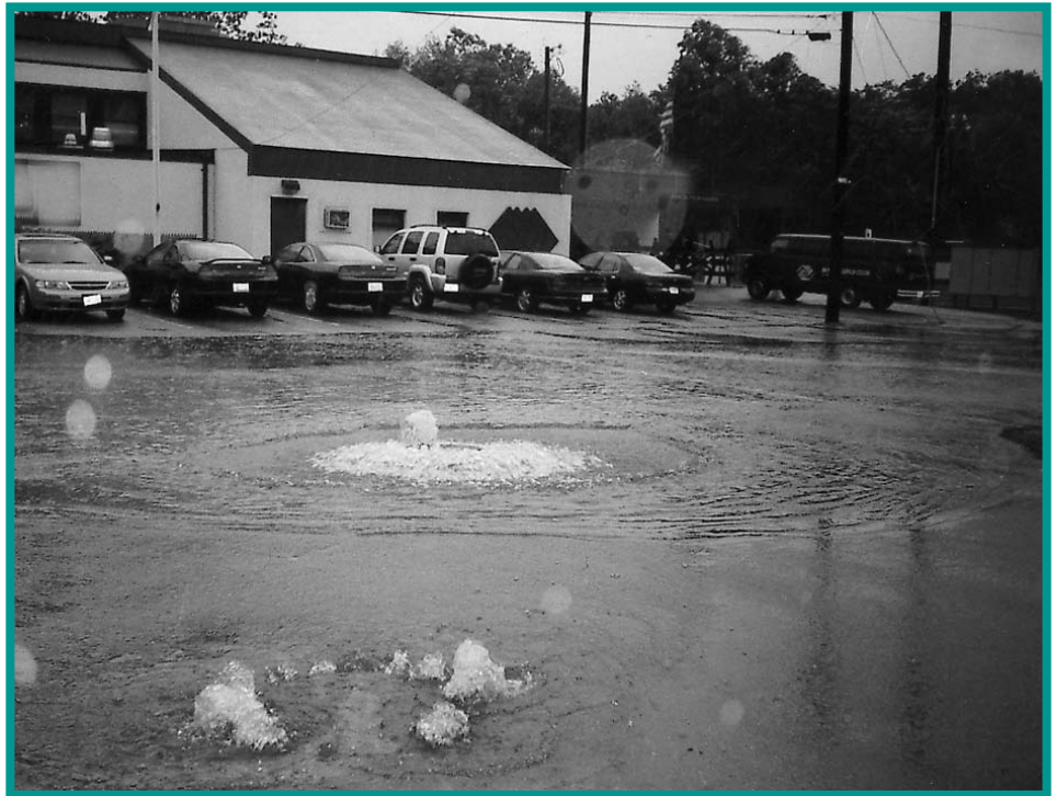
Two overflowing manholes flooding a street and parking lot in Rhode Island with contaminated water.
