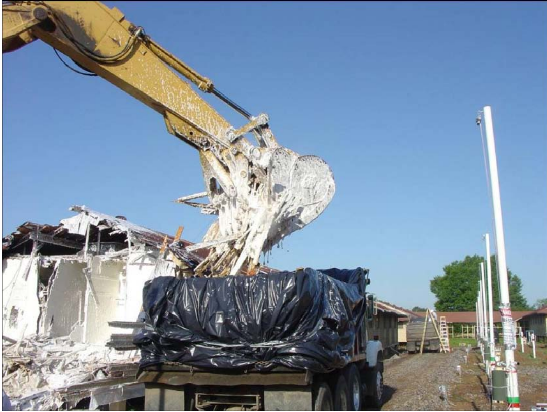
Figure 4-33. Loading the AACM demolition debris.
