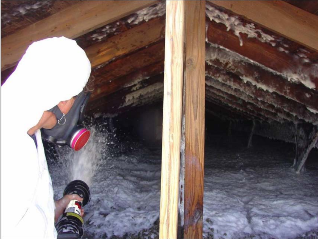
Figure 4-25. Pre-wetting the attic with Amended Water.
