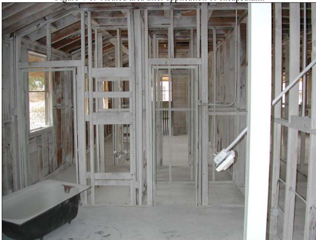
Figure 4-7. Abated area after final clearance.
