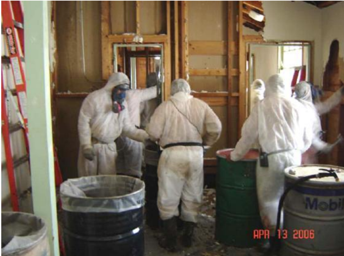
Figure 4-4. Loading abated material into barrels.
