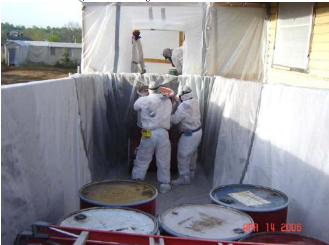
Figure 4-5. Loading asbestos-containing material into roll-off container.
