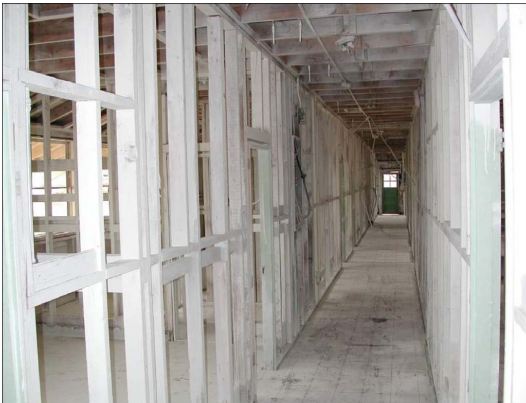
Figure 4-6. Abated area after application of encapsulant.
