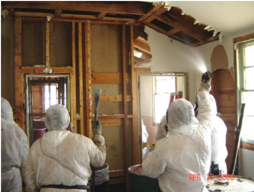
Figure 4-3. Wetting and removal of drywall during abatement of NESHAP building.
