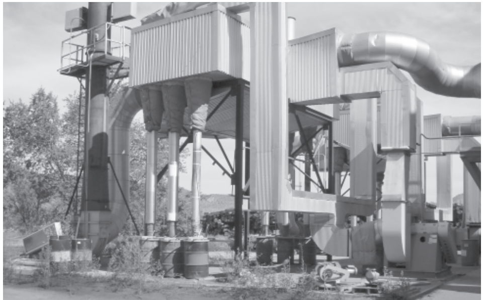
Collection of particulate matter from boilers at sawmill on Colville reservation.
