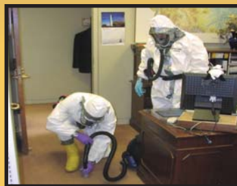
HEPA vacuuming the U.S. Senate offices to remove anthrax spores.
