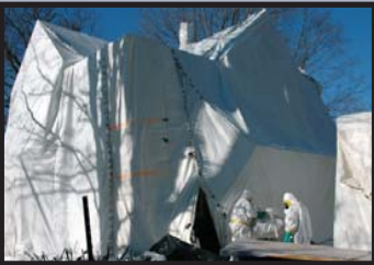
House tented for chlorine dioxide fumigation
