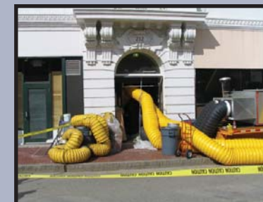
Heating up the building to improve remediation techniques.
