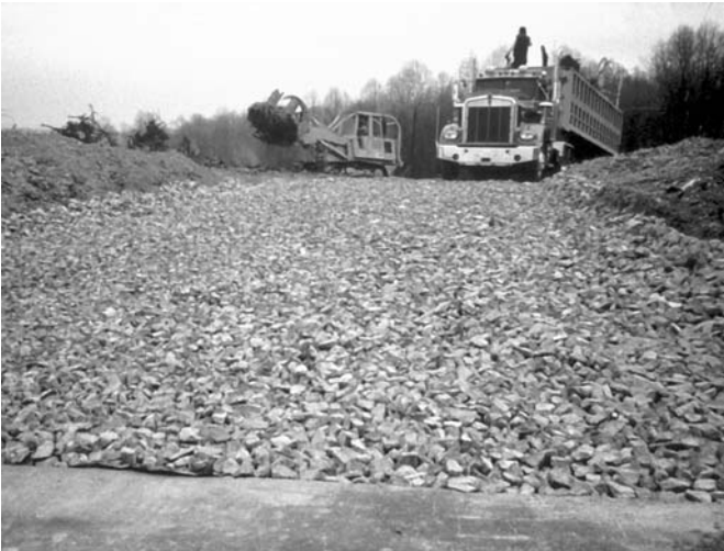
Stabilized construction entrances allow dirt to be removed from tire treads as trucks leave construction sites.
