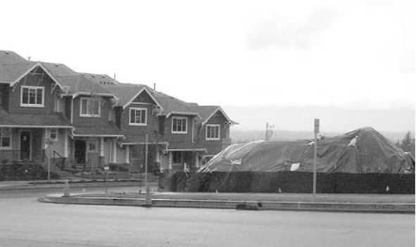
Covering dirt piles reduces storm water runoff velocity.
