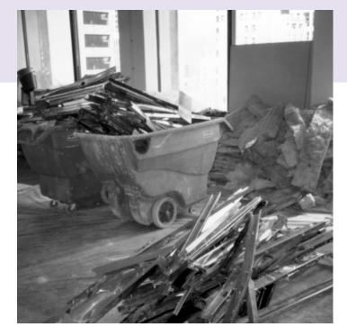
On site source separation of demolition materials was critical to a high diversion rate.
