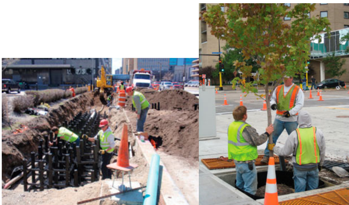
Figure 3-16. Under-sidewalk bioretention provides robust street trees as stormwater management benefit in the Minneapolis MARQ2 project.
