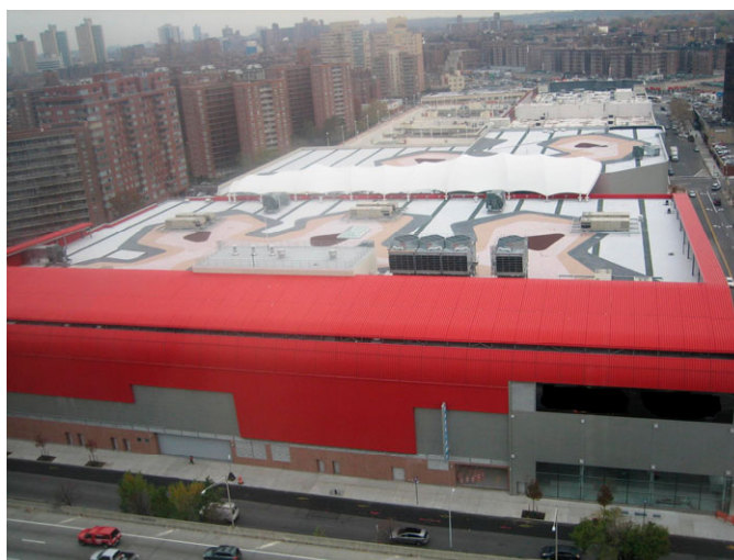
Figure 3A1-4. Rooftop detention being used to control runoff at a commercial property.
