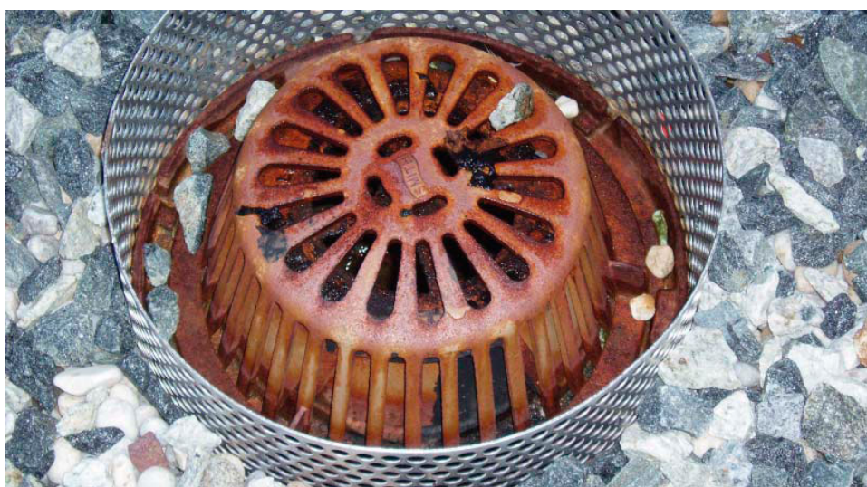
Blue roof drain installed by the SCA on PS 12 (Photo credit: Council on the Environment New York Source: Forester Media, Inc. www.Forester.net . Excerpted with permission.
