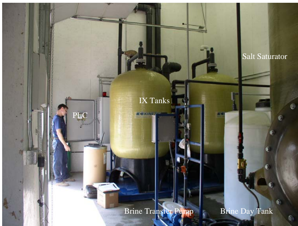
Figure 4-5. Photograph of IX-248-As/N System at Fruitland, ID
