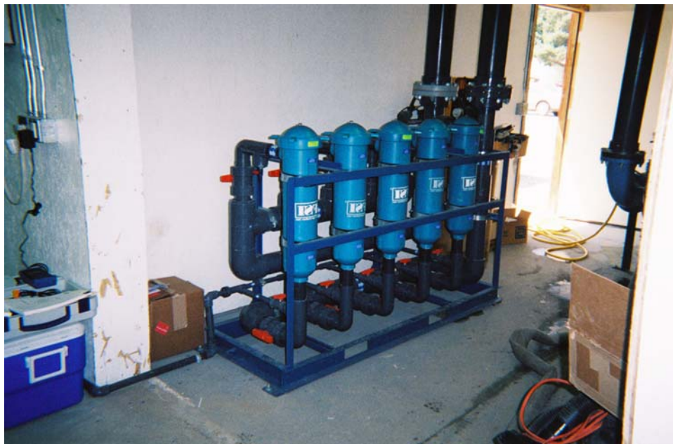
Figure 4-4. Photograph of Bank of Five Bag Filters
