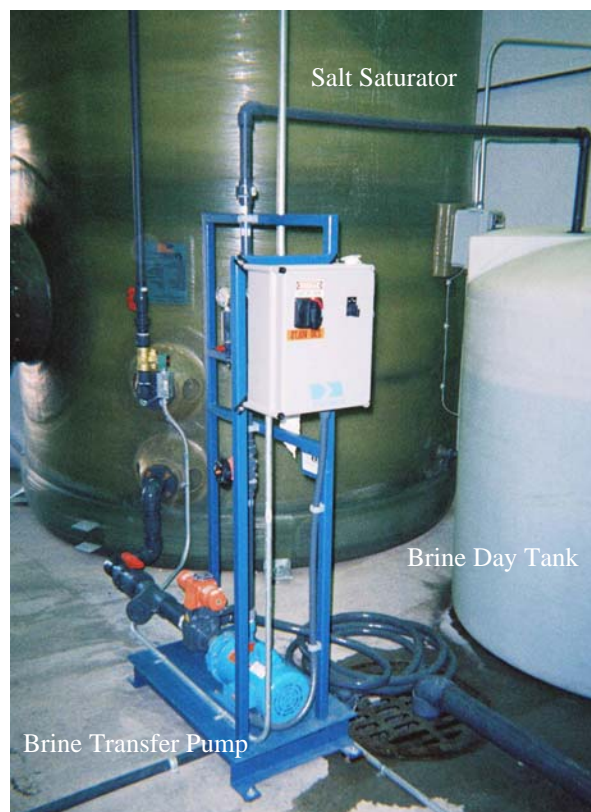
Figure 4-7. Photograph of Brine System
