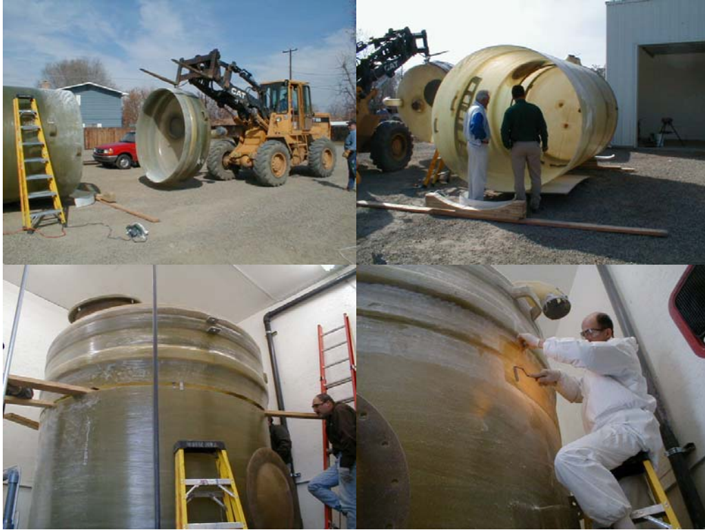
Figure 4-12. Cutting and Soldering Salt Saturator
