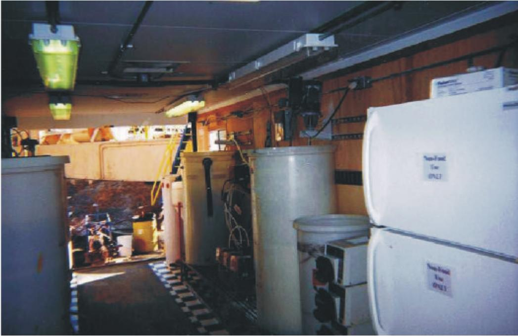
**Figure 1-5. Catalyzed cementation process in MWTP demonstration trailer.**
