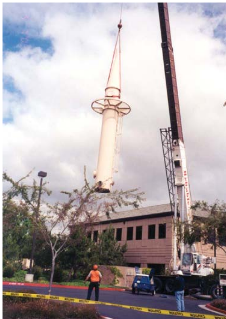
In Mountain View, Calif., responsible parties removed equipment that had treated TCE-contaminated groundwater by air-stripping, and replaced it with systems that release no TCE into the air.
