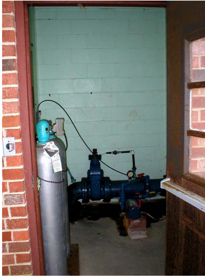
Figure 4-2. Chlorine Gas System at Well No. 1
