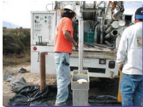
Drilling groundwater monitoring well.
