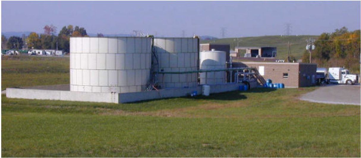
Photo 5: Sequential Batch Reactor (SBR) Leachate Treatment Facility
