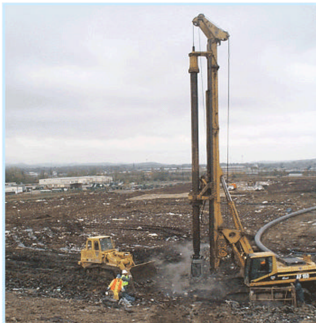
Photo 2: Drill Rig Equipped With a 3-foot Diameter Bucket Auger-Samples of Waste Are Collected in 10-foot Vertical Sections
