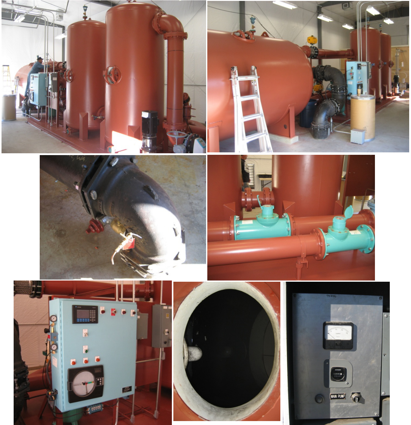
Figure 4-4. Treatment System Components (from left to right and top to bottom: Contact Tanks; Filtration Vessel; Sample Tap; Backwash and Effluent Flowmeters; PLC Control Panel; Filtration Media; Well Pump Controller and Hour Meter)
