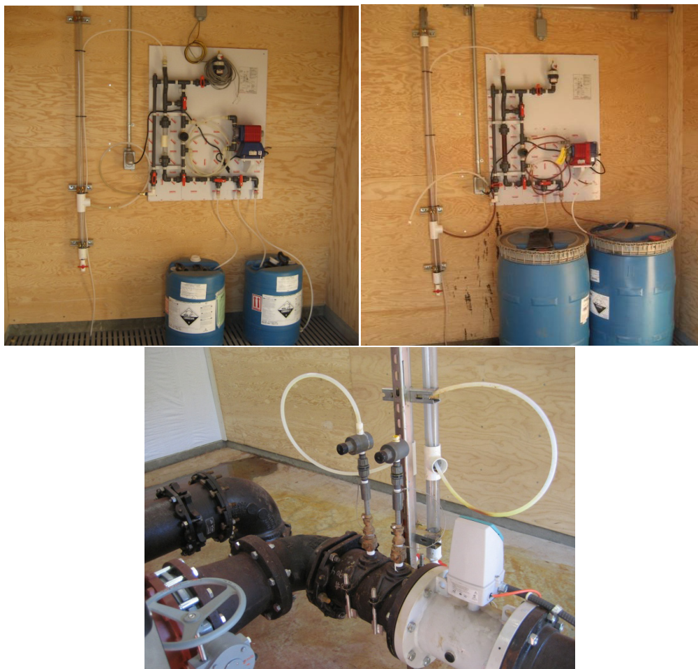
Figure 4-5. Chlorine and Iron Addition Systems (Clockwise from top left: NaOCl Addition System; Iron Addition System; NaOCl and Iron Injection Points)
