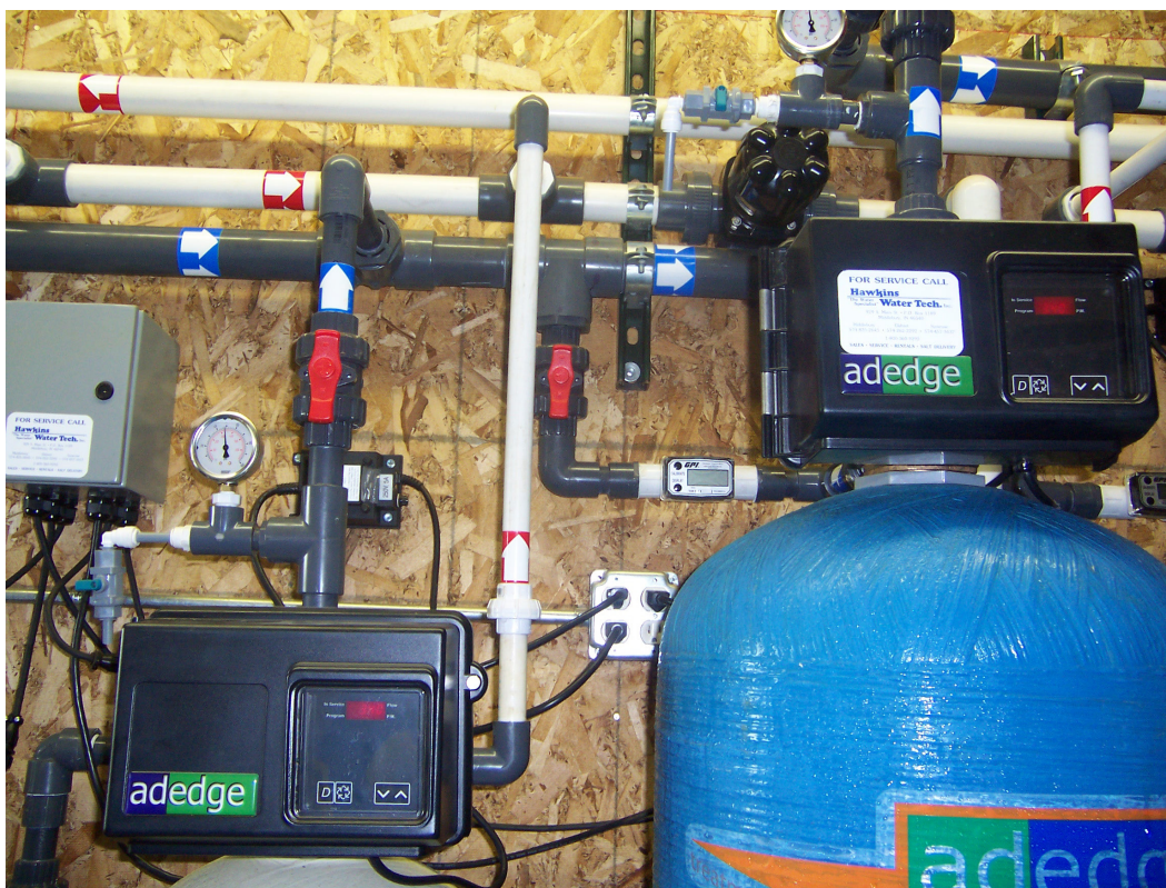
Figure 4-9. Fleck Controllers and Piping/Valves Connected to One AD26 (left) and One E33 (right) Vessel
