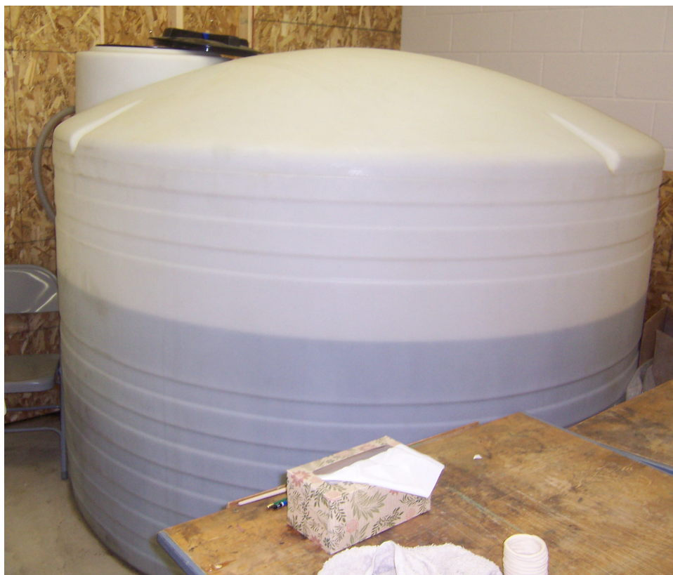
Figure 4-18. Temporary Storage Tank for Backwash Wastewater
