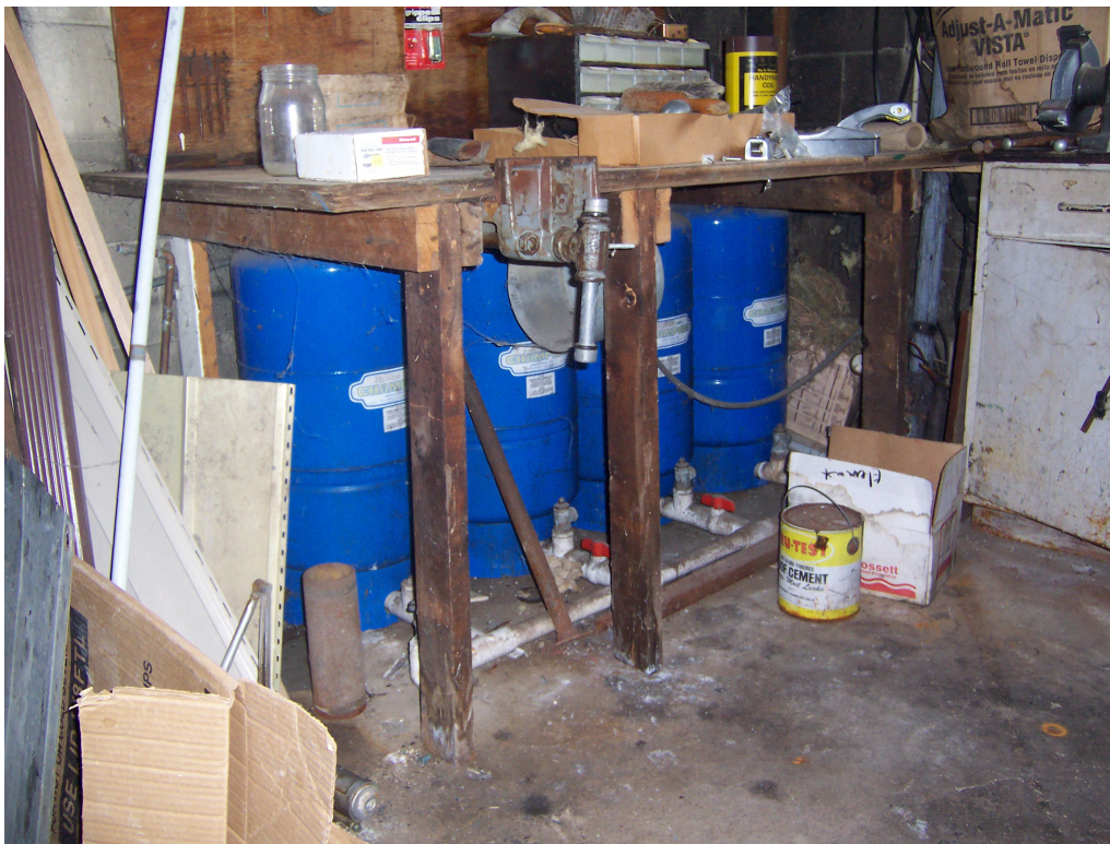
Figure 4-4. Pre-existing Water System Bladder Tanks
