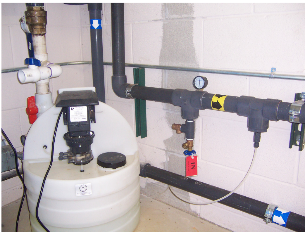
Figure 4-7. Chlorine Addition System
