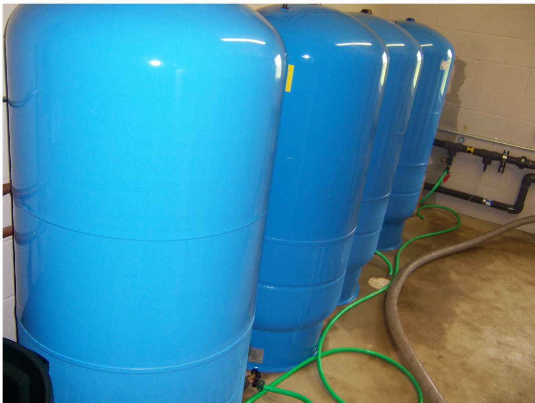
Figure 4-10. ProFlo PF119 Pressure Tanks
