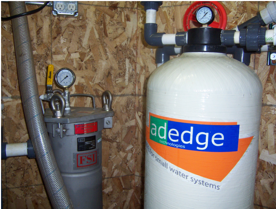
Figure 4-11. Bag Filter Assembly and GAC Tank
