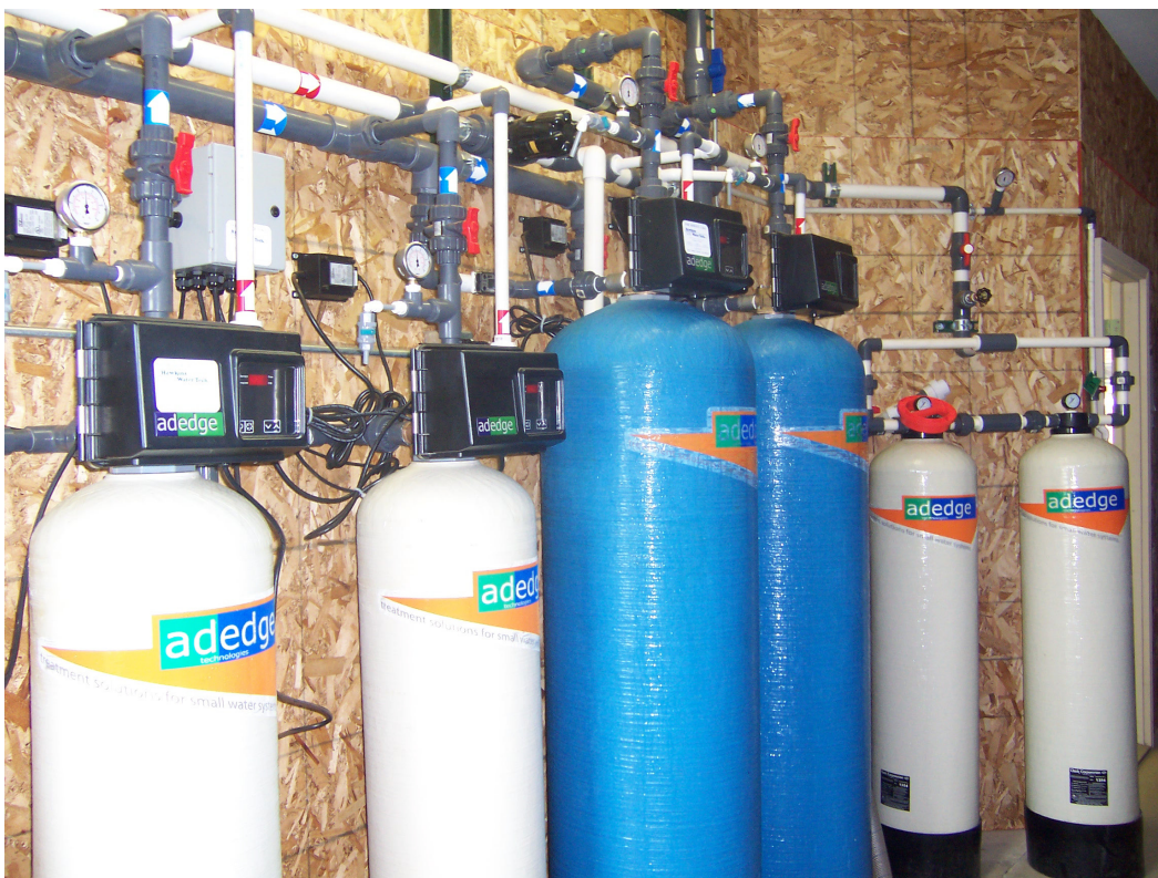
Figure 4-14. Treatment System Installed (From left to right: AD26 Vessels, E33 Vessels, and GAC Vessels; One AD26 Vessel and One Bag Filter Assembly not Shown)
