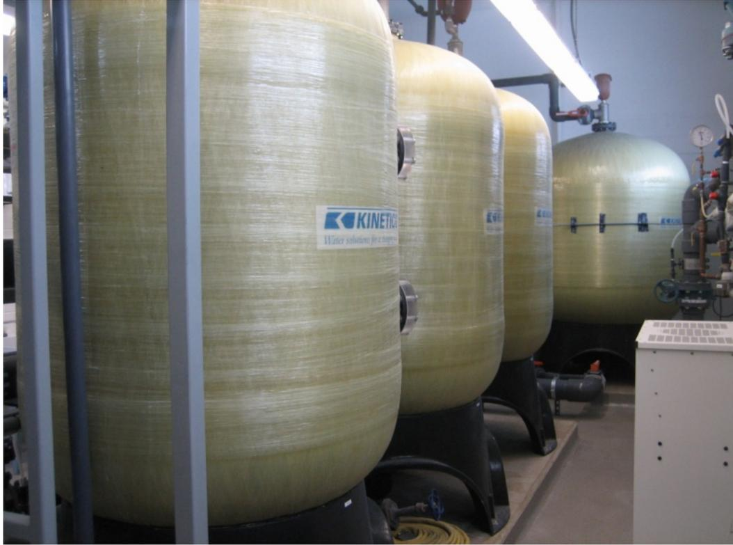
**Figure 1. Three Macrolite® Filters (foreground) and One Contact Tank (background)**
