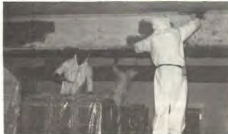
Removal of Wet Asbestos Material From Overhead Surfaces
