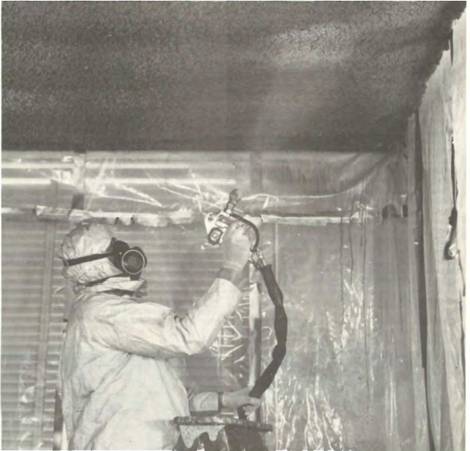
Encapsulation of a Ceiling Surface
