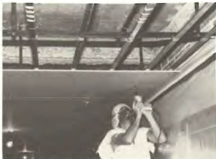
Constructing a Suspended Ceiling Barrier
