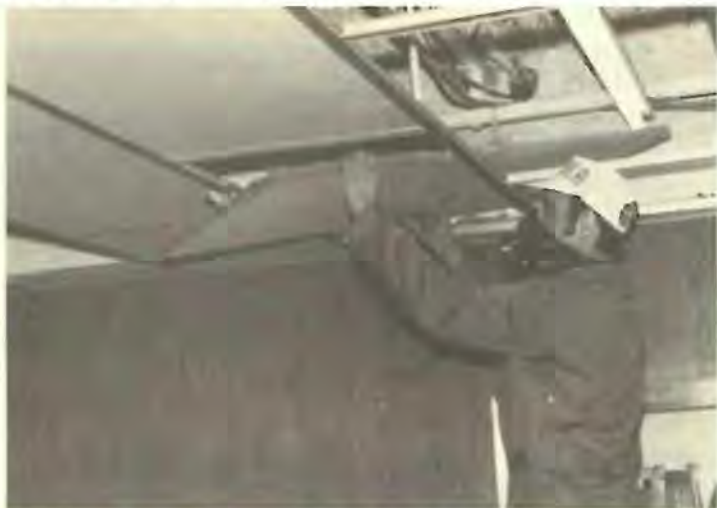
Removing Suspended Ceiling Panel For Inspection
