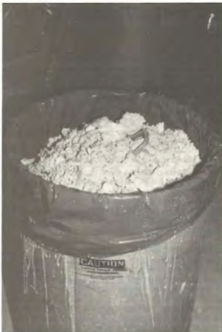
Removed Material in Drum With Plastic Liner
