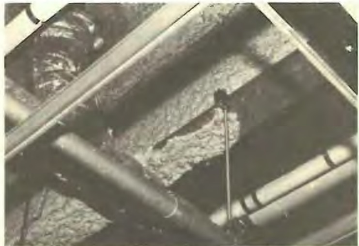
Area Above Suspended Ceiling With Friable Material
