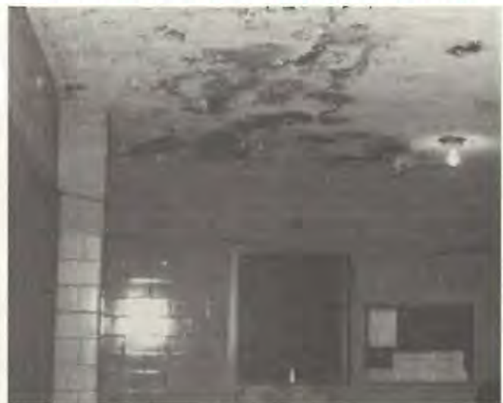
Friable Material Showing Water Damage
