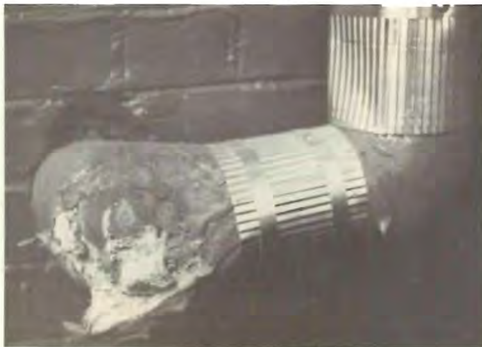
Damaged Pipe Covering Showing Friable Insulation Material
