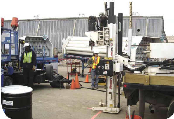
Pneumatic fracturing at the Hunters Point Naval Shipyard Superfund site
