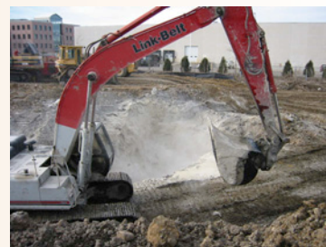
Sediment stabilization mixing operation
