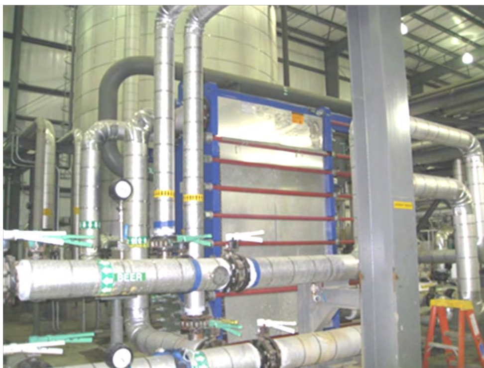
Figure 6.10. Heat capture through heat exchangers greatly improves energy efficiency in the Illinois ethanol plant.
