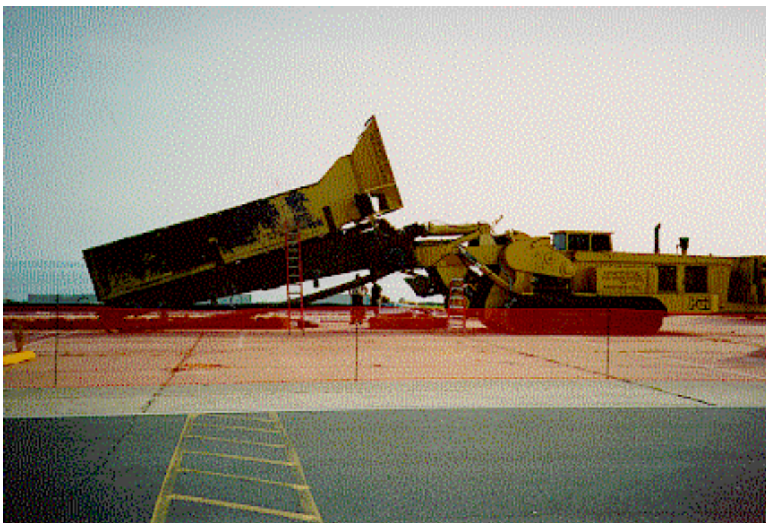
Figure 9. Continuous trencher used at Elizabeth City, North Carolina.
