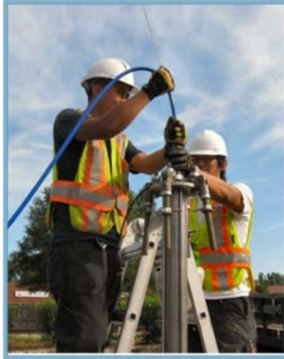
Technicians inserting the Sahara hydrophone into the pipe in live conditions.
