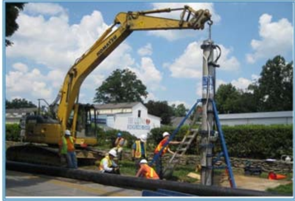
Setting up the PipeDiver extraction tube.
