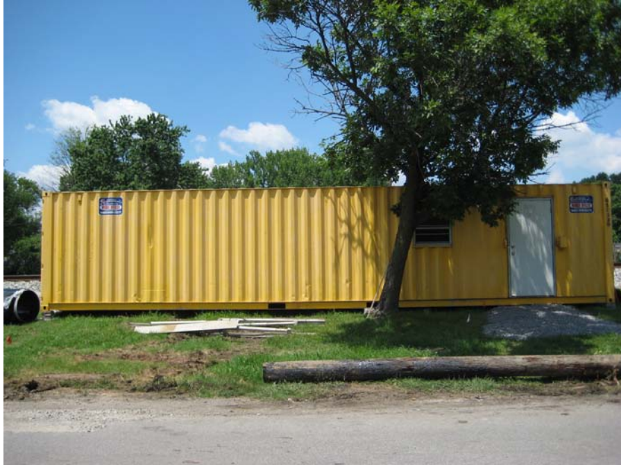
Figure 3-10. Construction Trailer for Equipment Storage and Work Space
