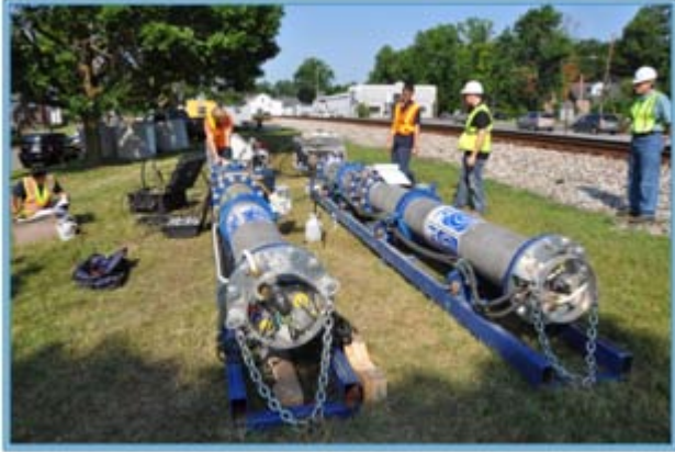
Preparing the PipeDiver insertion and retrieval tubes.
