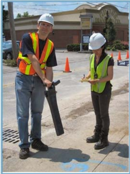
Technicians locating the PipeDiver vehicle from above ground.
