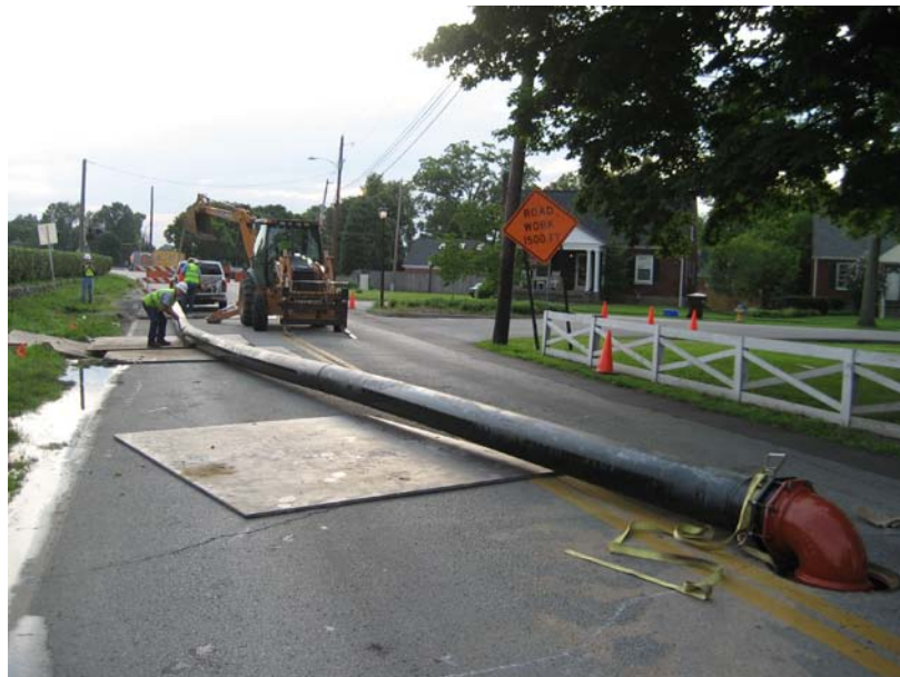
Figure 3-19. Test Pipe Discharge to Storm Sewer Configuration
