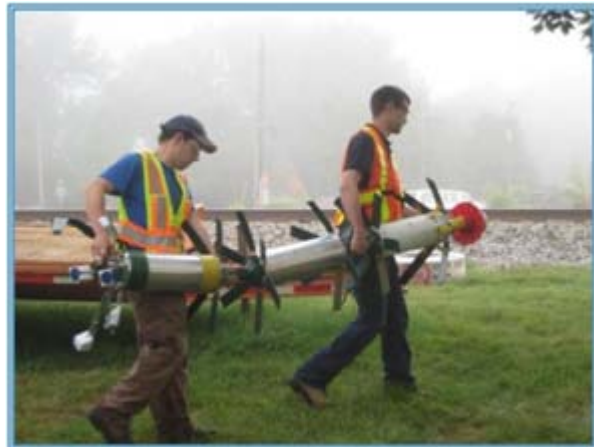
Carrying the PipeDiver tool ready to be installed into the insertion tube.
