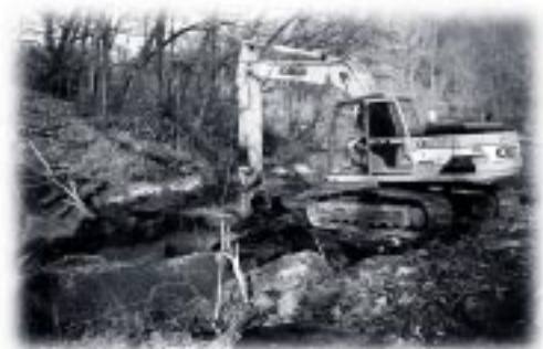
The Lititz Run Watershed Alliance in Pennsylvania removed an old dam to restore wildlife habitat and reduce thermal pollution in the stream.
