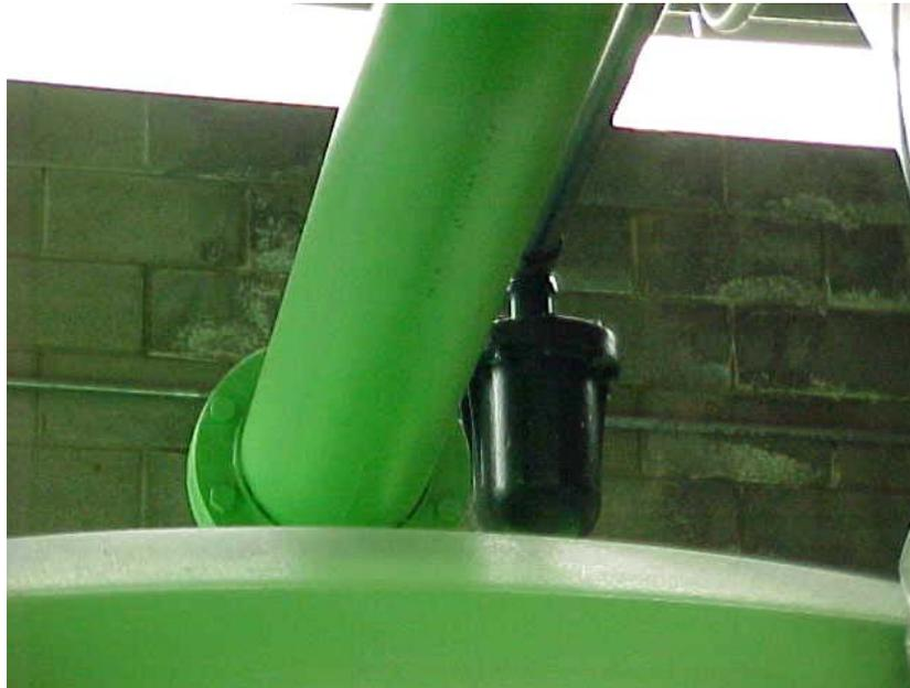
**FIGURE 5-4.** Air Release Valve
