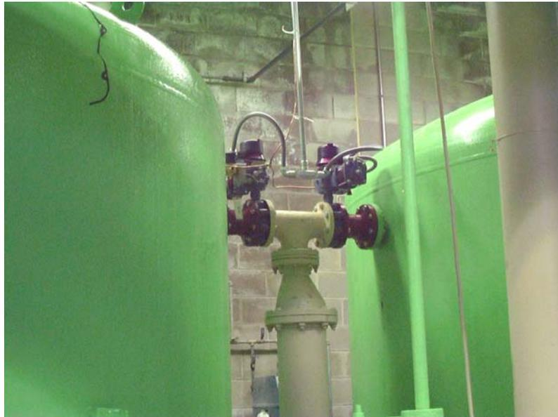
**FIGURE 5-8.** Pneumatically Operated Draindown Valves
