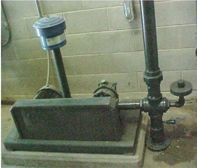
**FIGURE 5-5.** Air Wash Blower and Motor
