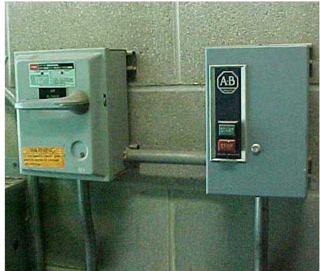
**FIGURE 5-6.** Air Wash Blower Controls
