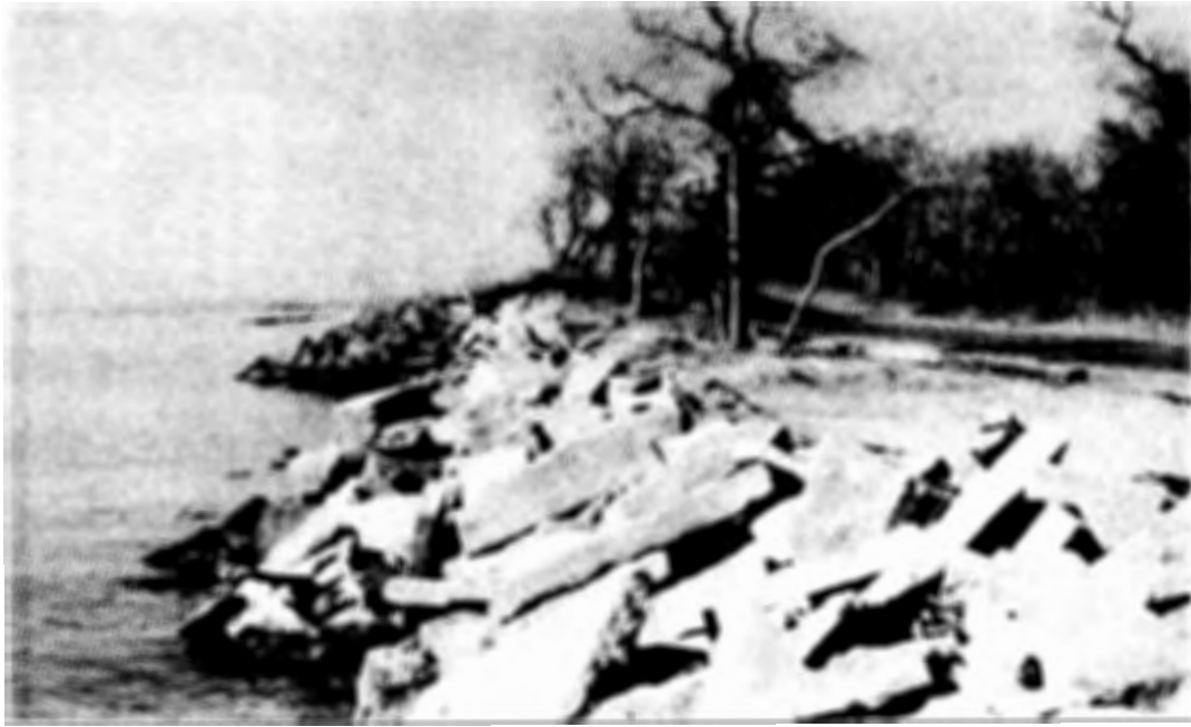
Figure 14. Rubble consisting of stone, demolished building and highways, and even junked cars, are often used to stop erosion, though the aesthetics vary.
