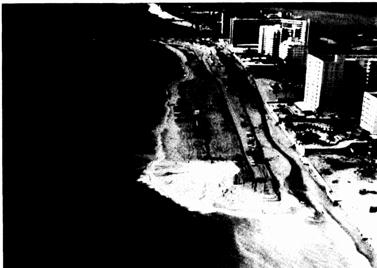
Figure 7. Beach nourishment along the Florida Atlantic coast is the preferred response to mitigate erosional problems and to maintain a wide recreational beach.
