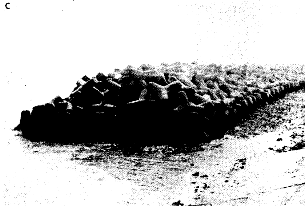
Figure 7. (A,B) Manual construction of seawalls to protect Male, capital of the Maldives. In the background of (B), a Japanese engineering firm manufactures tetrapods and builds a new breakwater (C).
