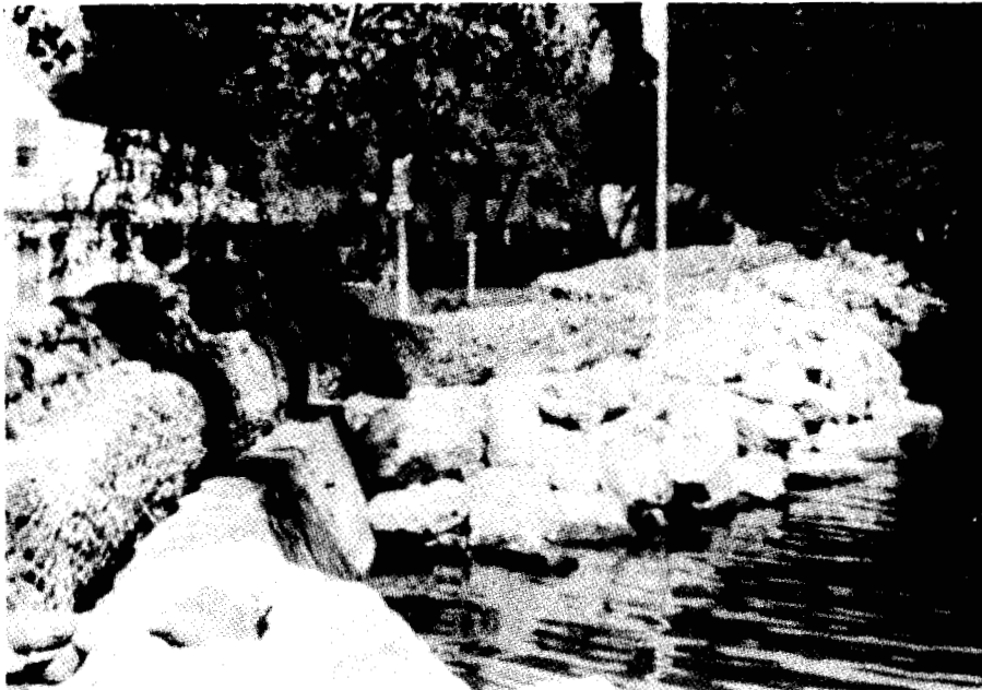
Figure 15. This home is protected by a stone revetment, wire baskets filled with stones, and sandbags.
