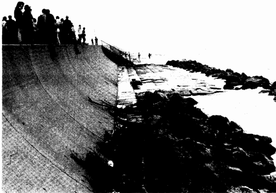
Figure 18. Although seawalls can protect property, the beach is eventually lost, as seen in Galveston, Texas (USA).
