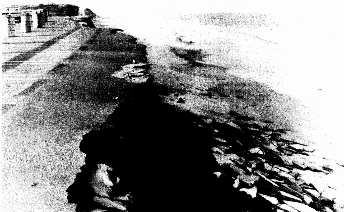
Figure 1. Continuing shore erosion threatens this parking lot at Coast Guard Beach, Cape Cod, Massachusetts. This is a national problem as best estimates are that about 90 percent of the U.S. sandy beaches are experiencing erosion.
