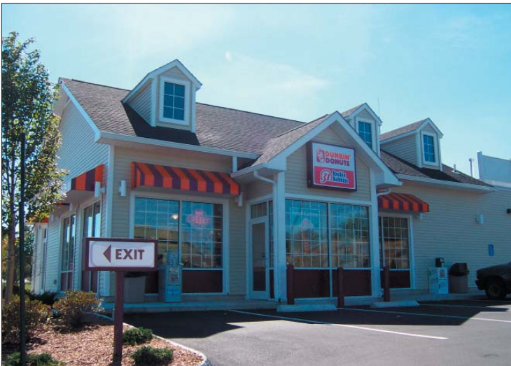
The Tinkham Garage site in reuse. Source: EPA
