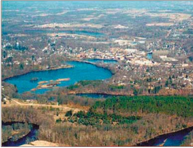
Aerial photograph of the Allied Paper, Inc./Portage Creek/Kalamazoo River area. Source: Michigan Department of Environmental Quality
