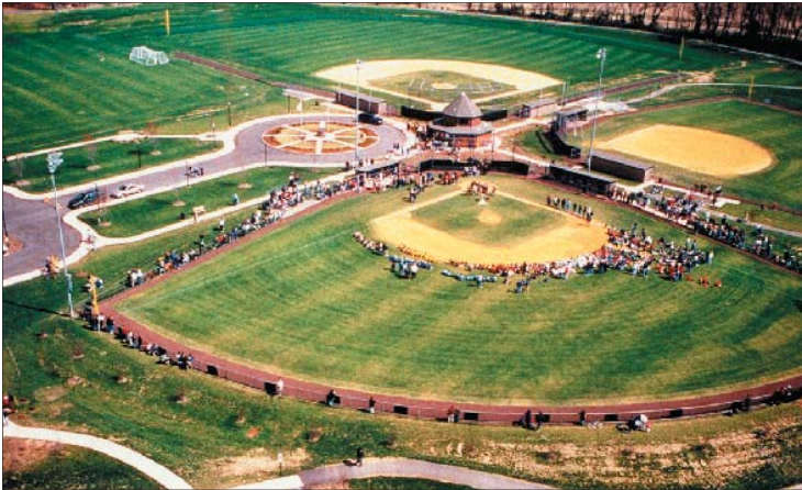
A sports complex, including six baseball and soccer fields, was built over waste containment areas at the Lipari Landfill Superfund site in Mantua Township, New Jersey. Source: EPA
