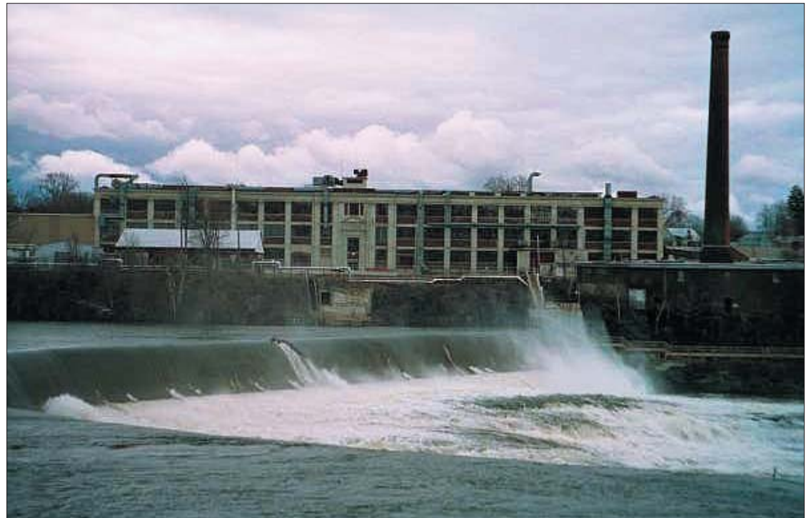
Hudson River PCBs site in New York where the group Scenic Hudson, Inc. used TAG funds to keep the community in Ft. Edward informed through newsletters and a Web site about the river cleanup. Source: EPA
