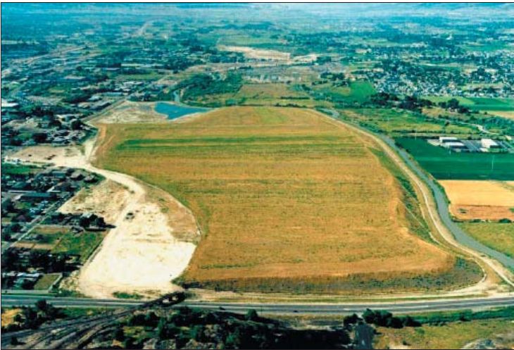
Sharon Steel as it is today, ready for redevelopment. Source: EPA
