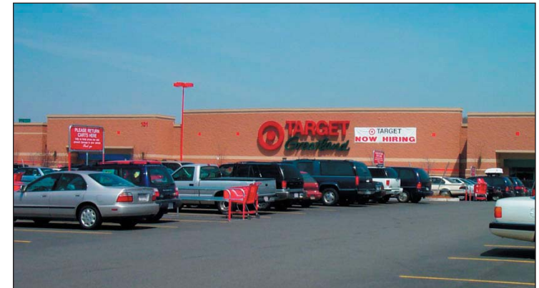
Target at the Industri-Plex Superfund site. Source: EPA
