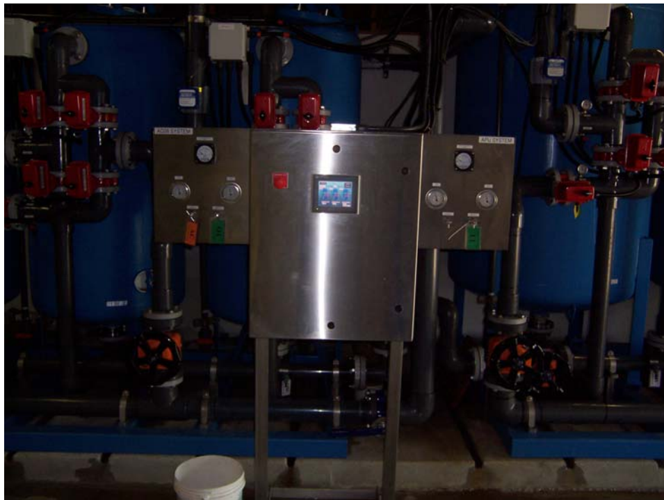
Figure 4-10. System Control Panel
