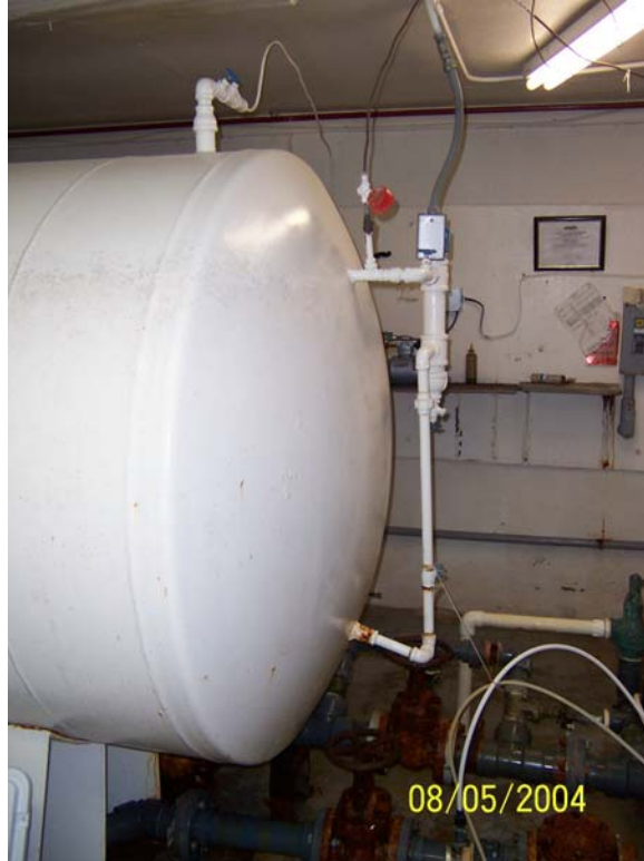
Figure 4-3. Pre-Existing Storage Tank
