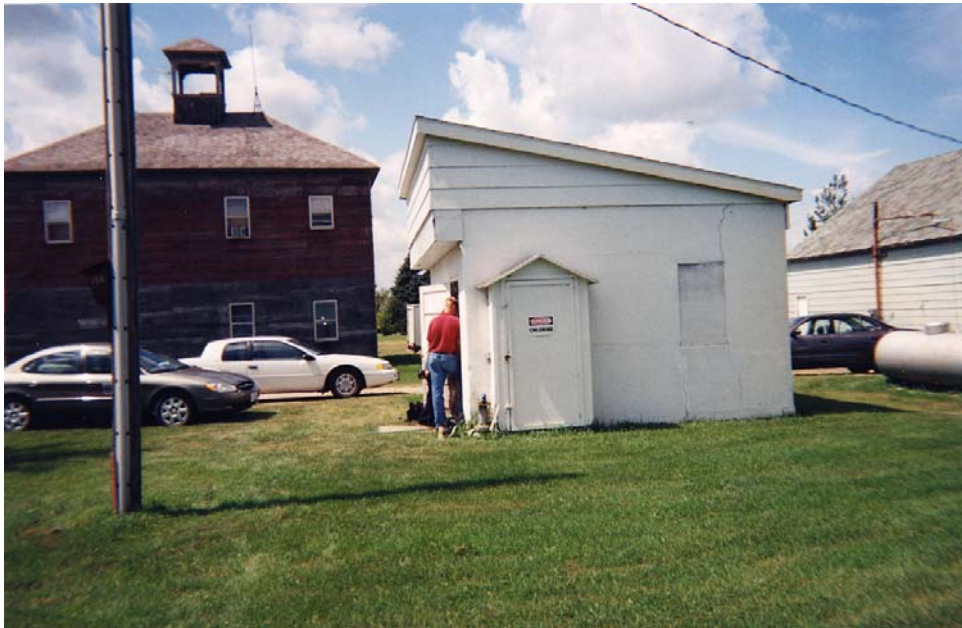
Figure 4-1. Pre-Existing Pump House at Climax, MN, Site
