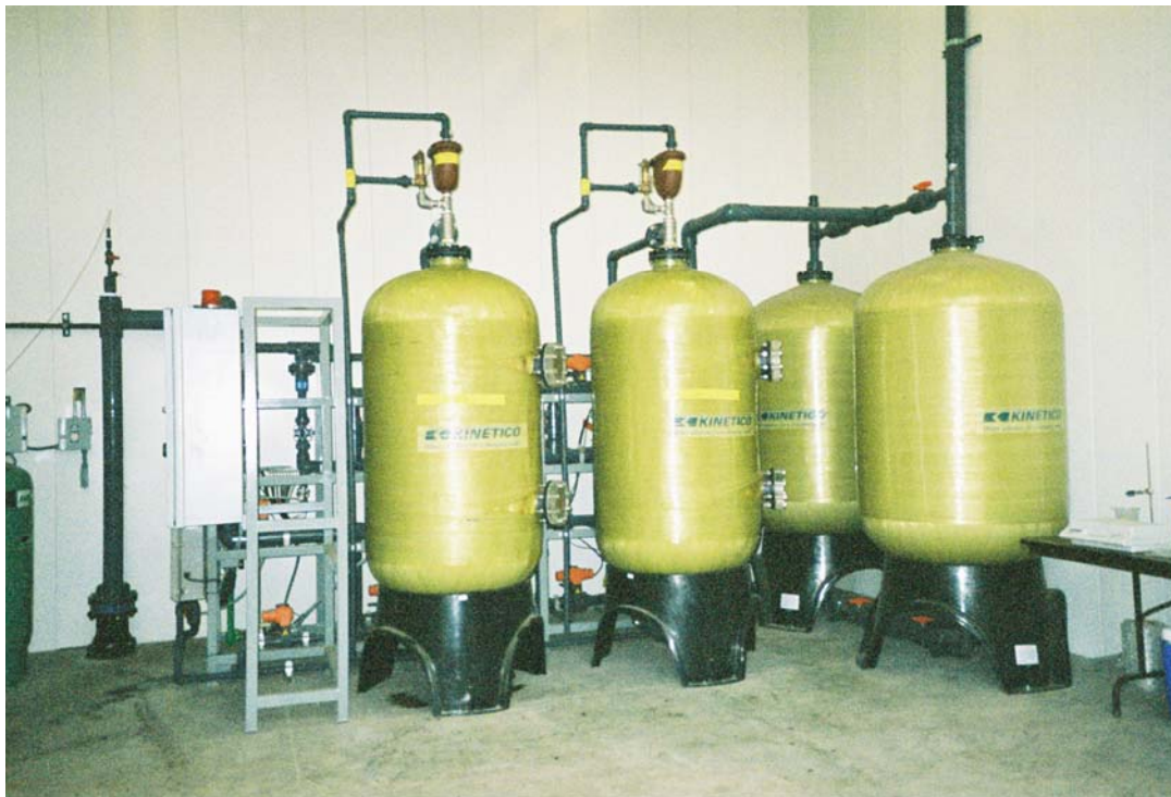
Figure 4-5. Photograph of the Macrolite® Pressure Filtration System
