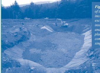
Figure 3. Construction of the Ore Hill BCR, including sediment excavation, lining installation, plumbing, and reactive substrate placement, was completed within a single month.
