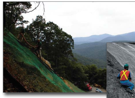
Figure 9. Netting stabilizing a compost blanket
