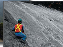
Figure 10. Stapling netting to the slope
