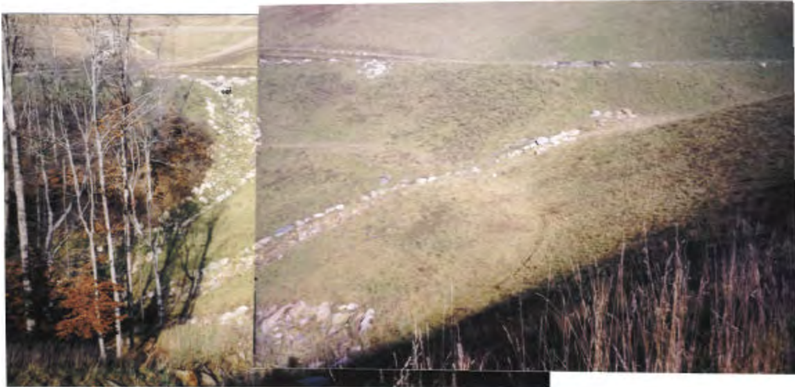
Groin ditches convey storm flow down face of valley fill
