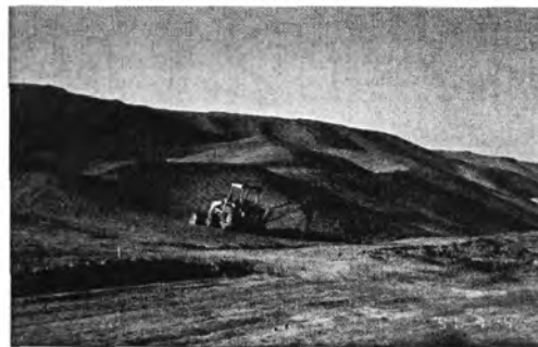
As opposed to the rigid forms of conventional grading (below left), landform grading (below right) provides shadows, depth and a more natural looking hillside.
