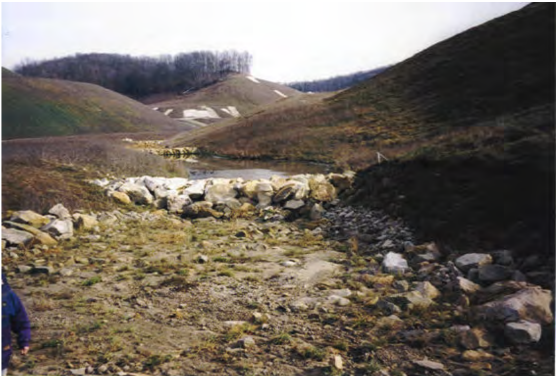
Outfall of combination ditch. Baseflow has gone subsurface into valley fill.
