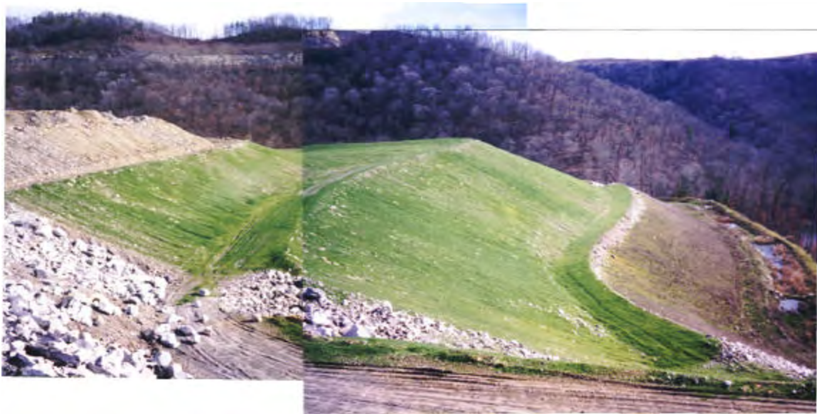
Active valley fill with perimeter ditches across face of fill.
