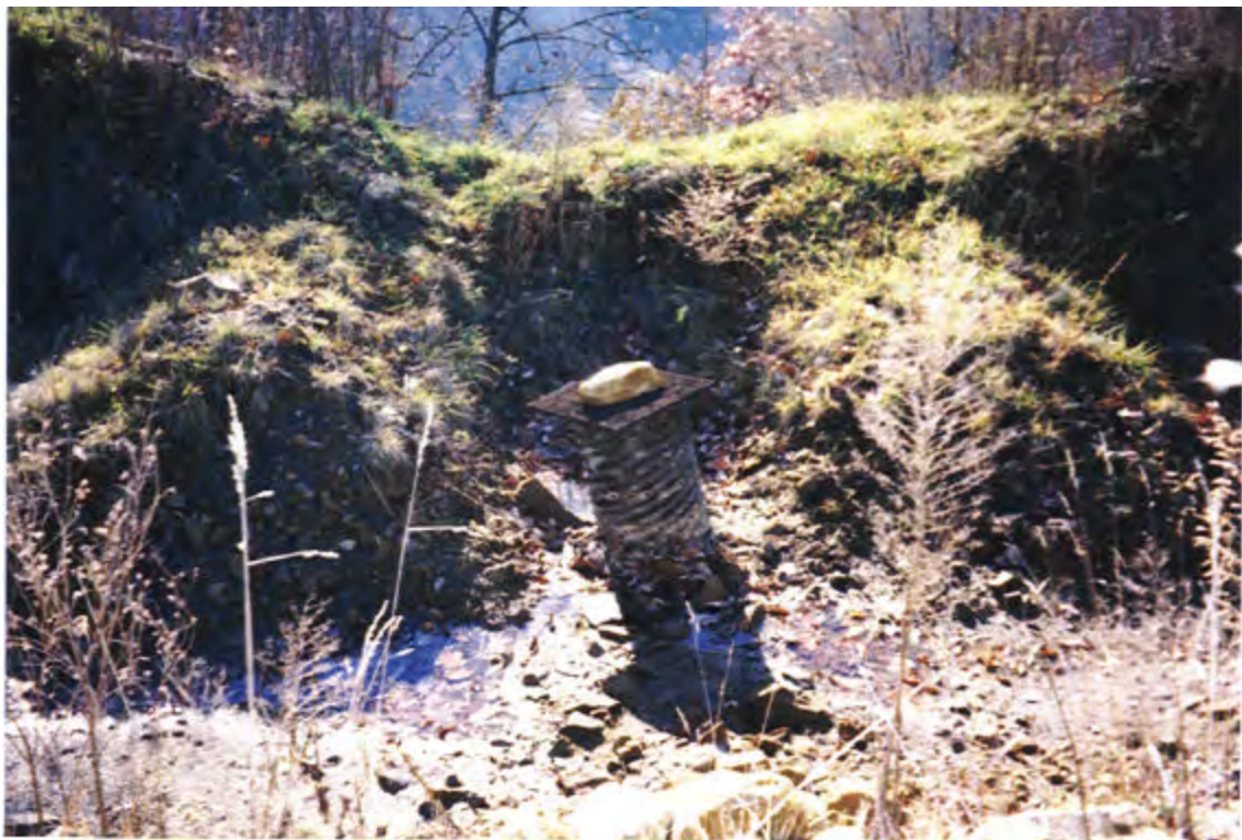
Outfall control structure for sedimentation ditch
