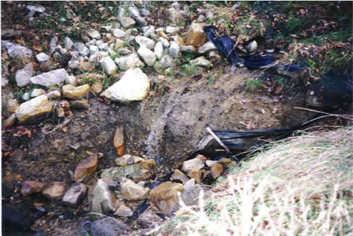
Headcut erosion at break in slope at downstream end of runoff ditch
