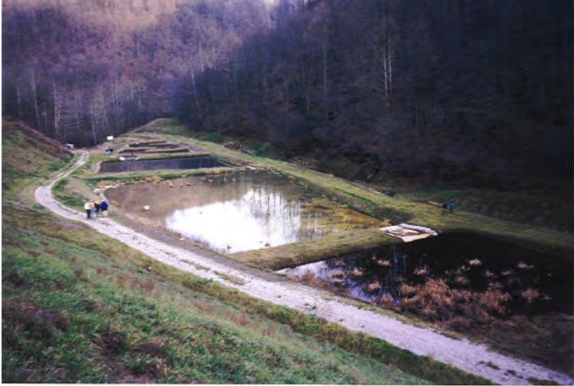
Wetland ponds downstream of sedimentation pond. Photo shows runoff ditch to right of wetland ponds. This ditch conveys baseflow and stormflows.
