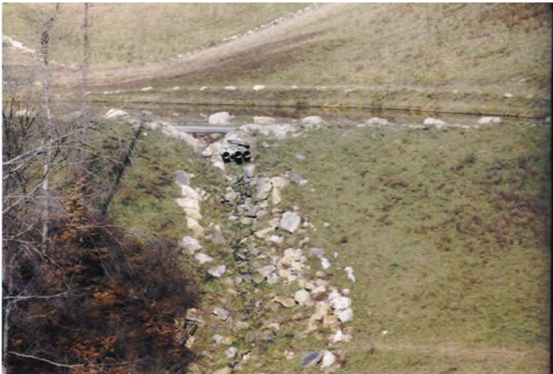
Groin ditch from upper sedimentation pond. Photo shows outfall pipes from pond and early evolution of "natural" channel within ditch.
