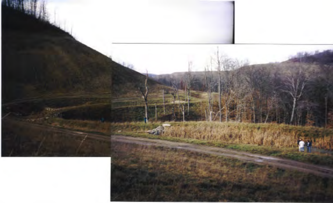
Combination ditch with baseflow supporting wetland vegetation
