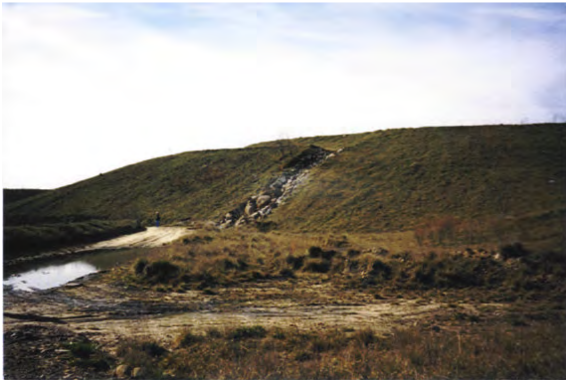
Older (pre-1994) reclaimed area. Valley fill with groin ditch to perimeter ditch.
