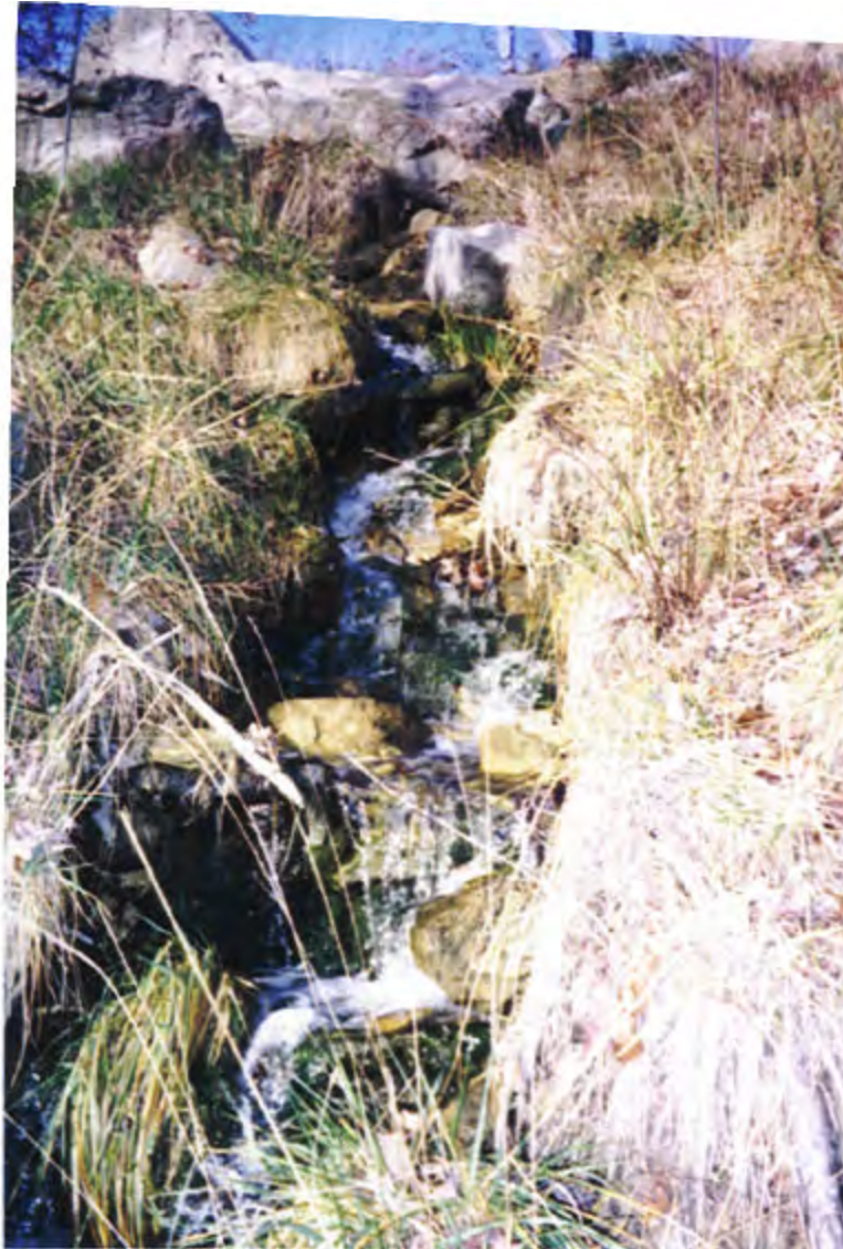
Outfall of combination ditch routed over undisturbed forested hillslope
