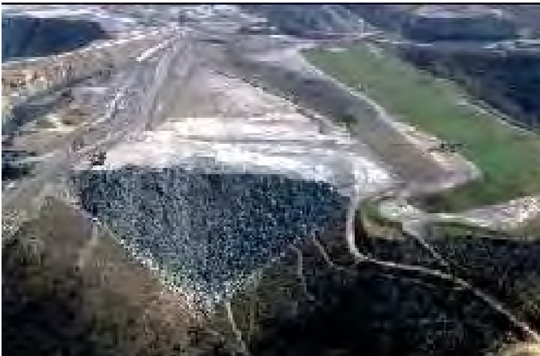
Figure 1-2. A VF in operation. The excess materials from a MTM operation are being placed in this adjacent valley.
