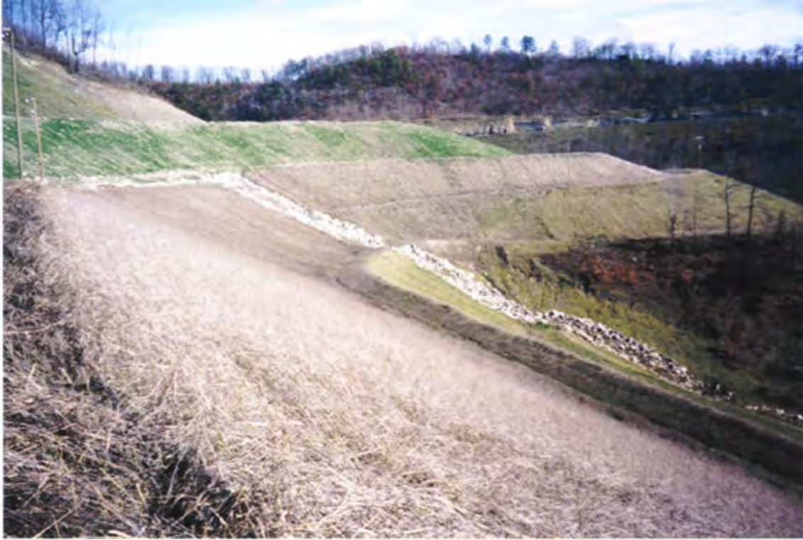
More recent (post-1994) reclaimed area. Valley fill with perimeter ditches and groin ditches to convey runoff from slopes.
