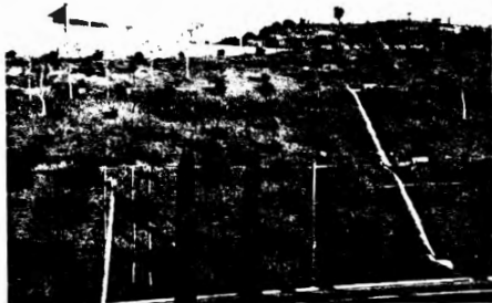
FIG. 2. Conventionally Graded Hill Slope with Planar Face, Rectilinear Drainage Ditch, and uniformly Spaced Plantings
