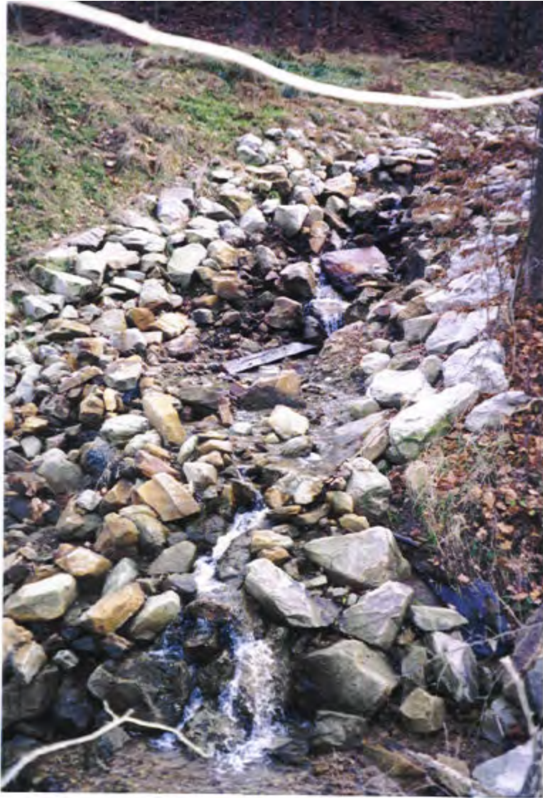
Headcut erosion working upstream through steep section of runoff ditch
