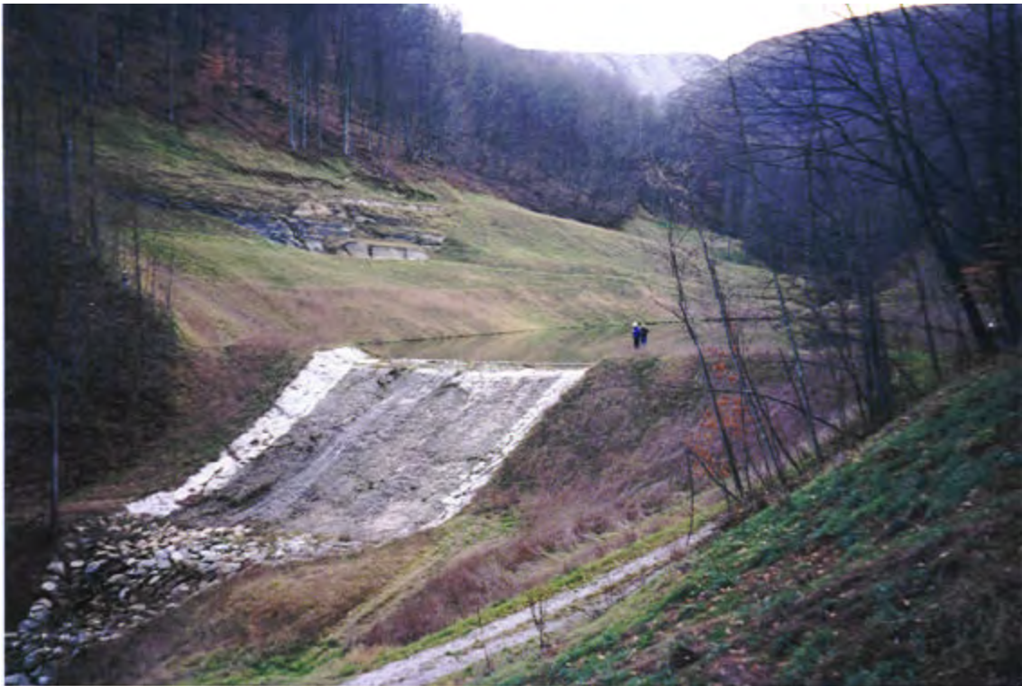
Concrete spillway of on-line sedimentation pond
