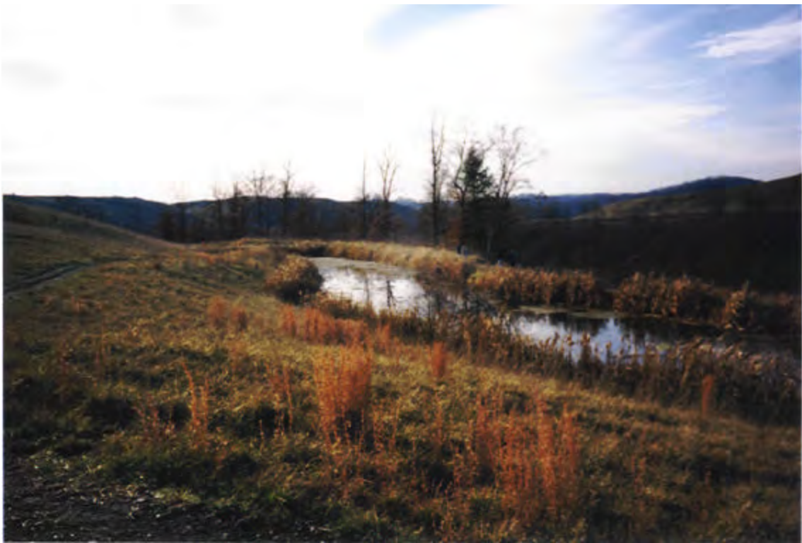
Combination ditch with baseflow. Photo shows wetland vegetation along margins of ditch.
