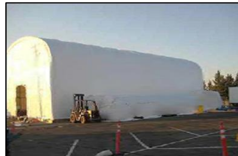
Figure 1. Two story building, without and with secondary containment (tenting), at Idaho National Laboratory.
