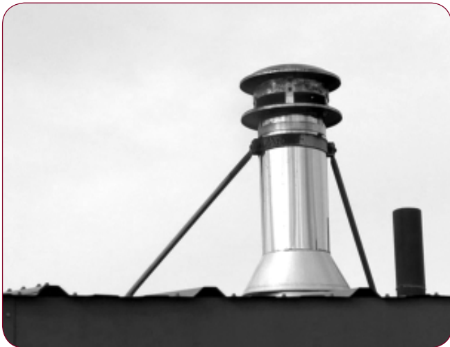
A clean burning wood stove with no visible smoke.
