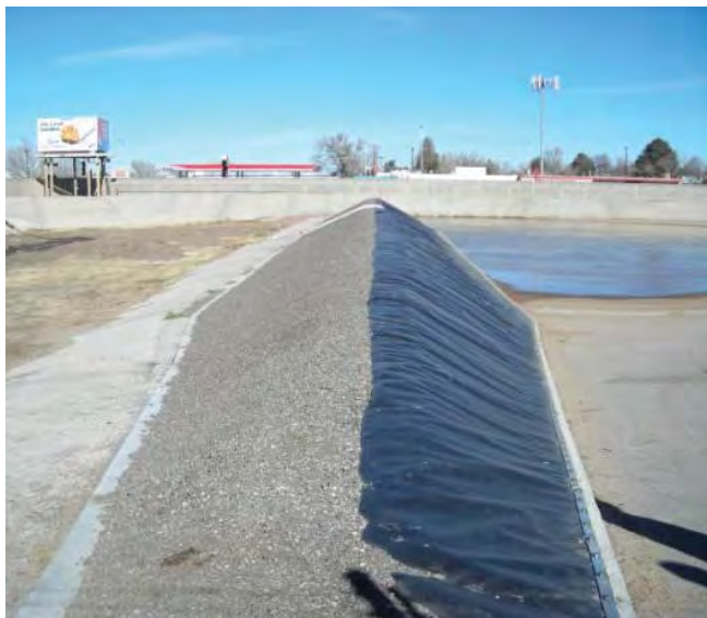
Photo 6. Dam to separate storm water runoff from city streets and runoff (process wastewater) from the CAFO production area. The left side is the storm surge pond used to store runoff from city streets. The right side is the CAFO wastewater retention pond.
