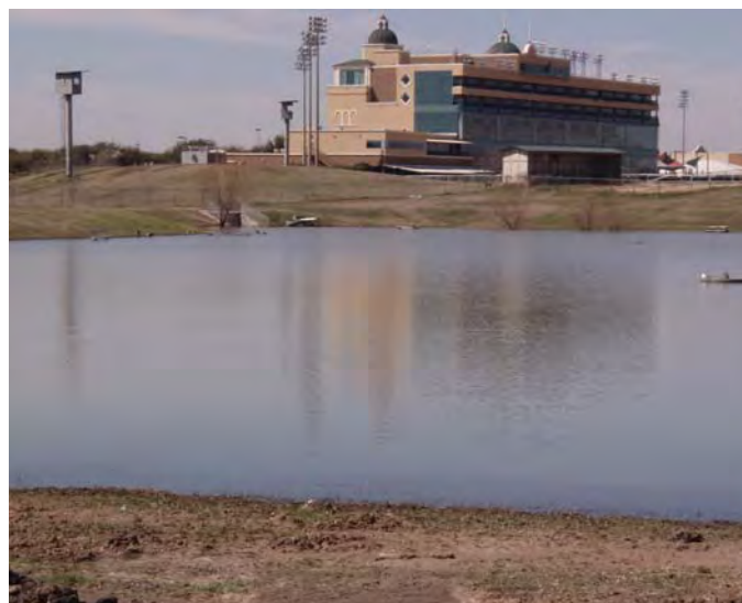
Photo 11. Retention control structure for storage of storm water runoff from the horse barns, horse paths, and manure storage areas/barns.
