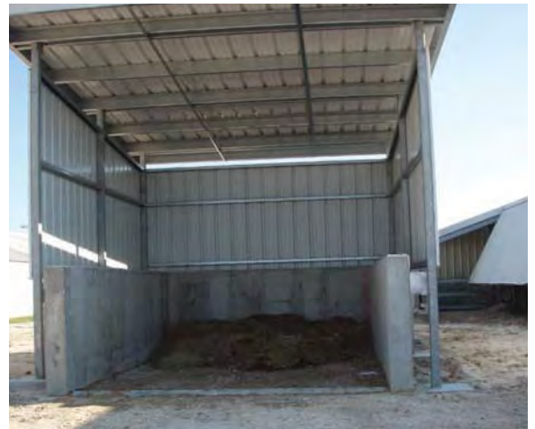
Photo 5 (right). Modified manure storage bin with extended walls and a roof to minimize contact with storm water.
