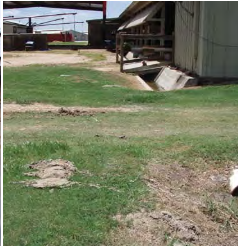
Photo 2. Wash rack drainage ditch.
