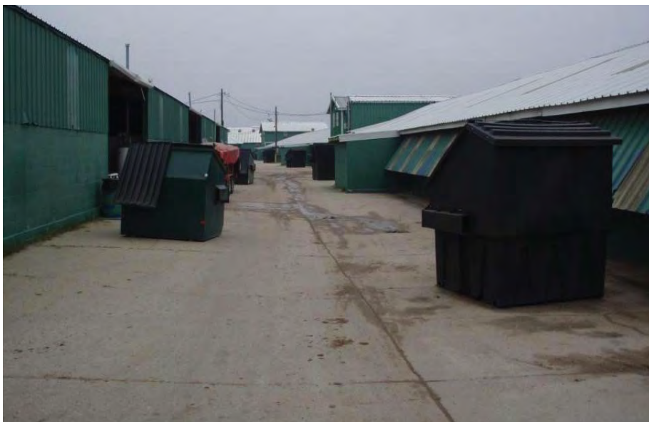
Photo 9. Old and leaking steel dumpsters for horse manure storage.
