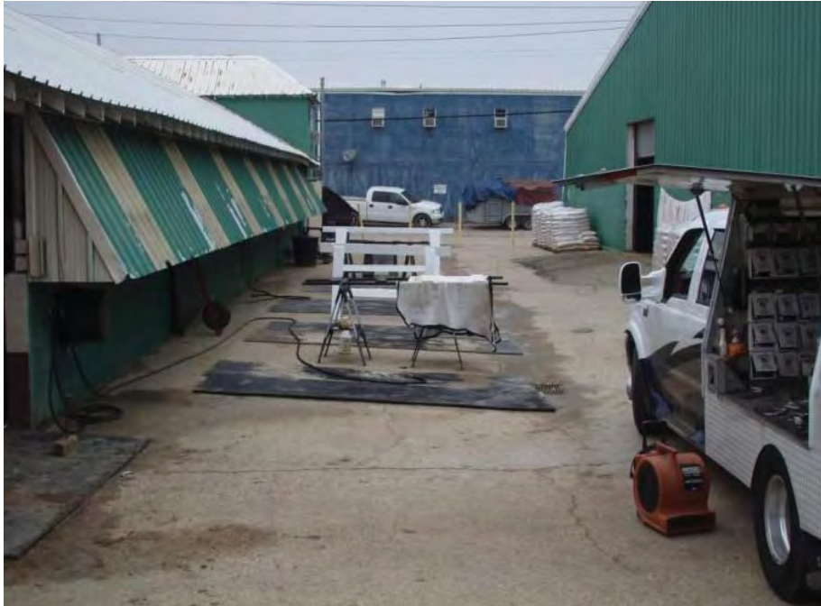
Photo 8. Uncovered horse wash rack located between barns.
