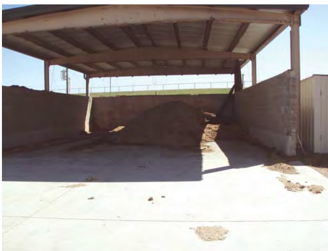
Photo 12. Covered and concrete-lined manure storage barn.
