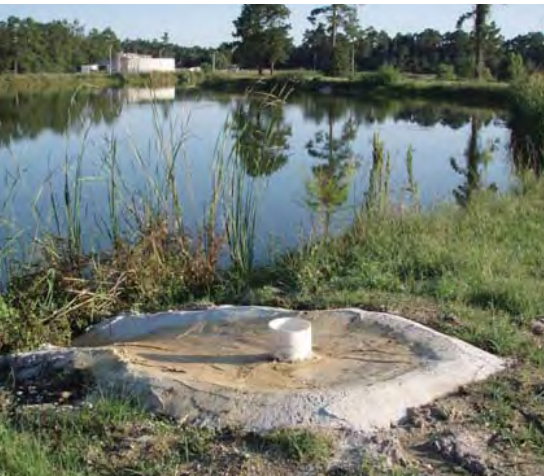
Photo 4 (left). All the horse wash water generated from covered wash racks is collected and pumped into a properly designed lagoon.
