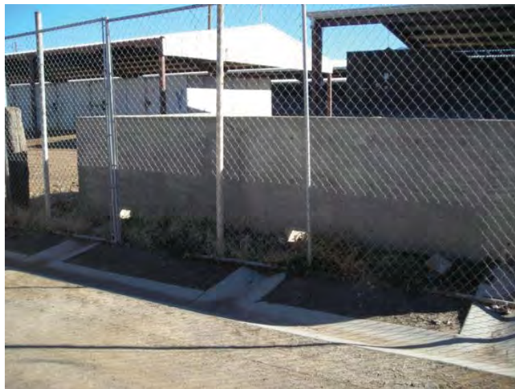
Photo 7. Covered horse wash rack connected to a concrete-lined wastewater conveyance system.
