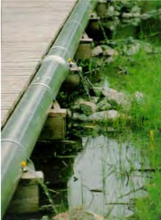
*Aluminum pipes distribute the treated effluent.*
