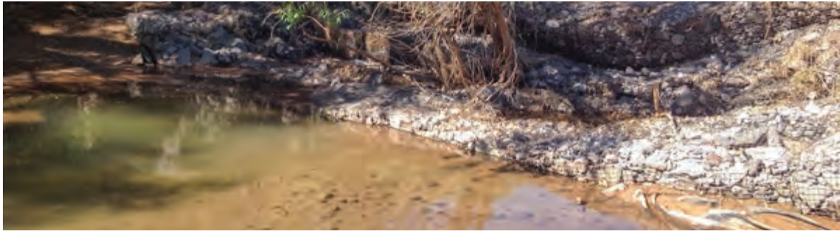
Water-harvesting gabion stabilized by downstream cottonwood, post-hurricane Odile, October 16, 2014. Source: Arizona Department of Environmental Quality
