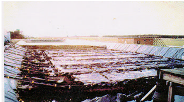
Figure 6 Lagoon based remediation of dredgings (Source: Geokinetics, International, Inc., Electrokinetic Remediation of Toxic Metals: Statement of Qualifications , June 1997)
